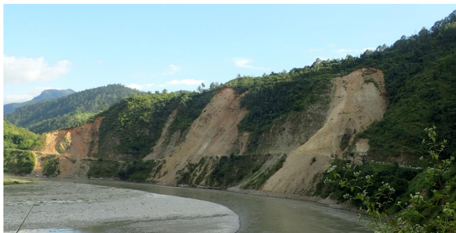
Figure 17.2-2 Collapse of Roadside Slope and Temporary Traffic at the Mid-Hill Highway
