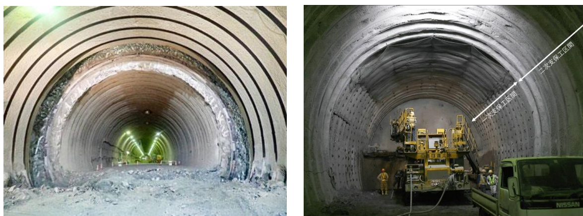
Figure 17.3-3 Outline of Multiple Support System
