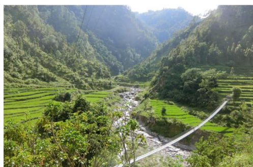
View to opposite direction form portal
