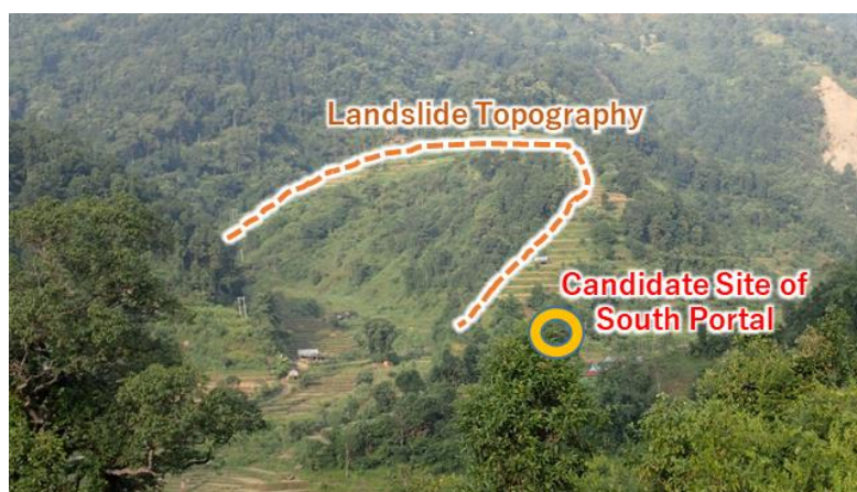
Figure 13.2-10 Landslide topography located near the proposed south tunnel portal
