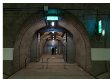
Evacuation Route (Evacuation Connection Tunnel)
