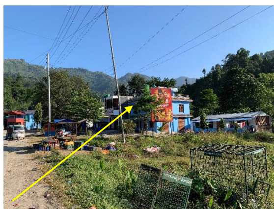
An image of designed alignment of the approach road separated from the existing road to a residential area
