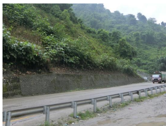
(b) Retaining wall
