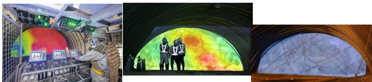
Figure 17.3-6 On-Site Visualization of the geological information on the cutting face
