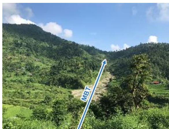
Figure 13.3-4 MBT line crossing the south portal
