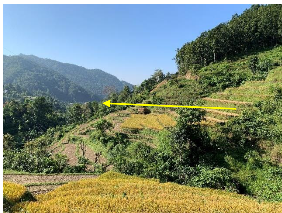
An image of the portal location at the middle of hillside (Alternatives in the right bank)
