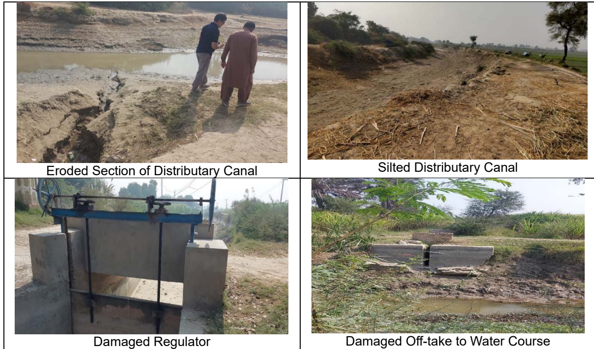
Figure 5.2.4 Current Condition of Distributory Canal
