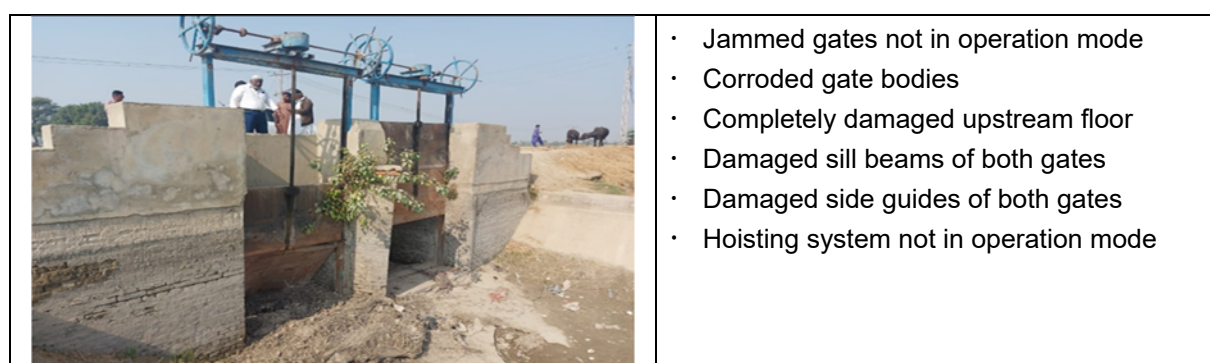
Figure 5.2.3 Current Condition of Off-take at the Head of Ali Bahar Distributary Canal
