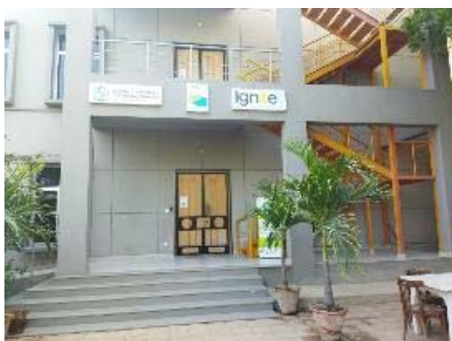
One of the facilities of NIC Karachi
