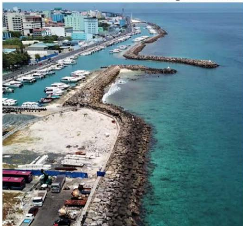
New shipping channel and stone seawall
