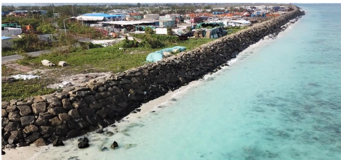
On the north coast, stone seawalls sufficient for coastal protection have already been completed.
