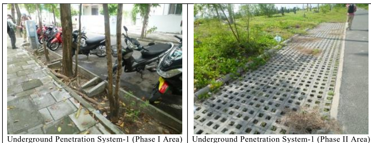
Figure 3-2.6 Rainwater infiltration facilities on Hulhumale Island
