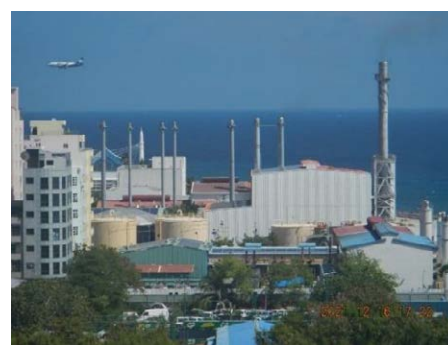
Figure 3-3.2 Thermal power plant at STELCO
