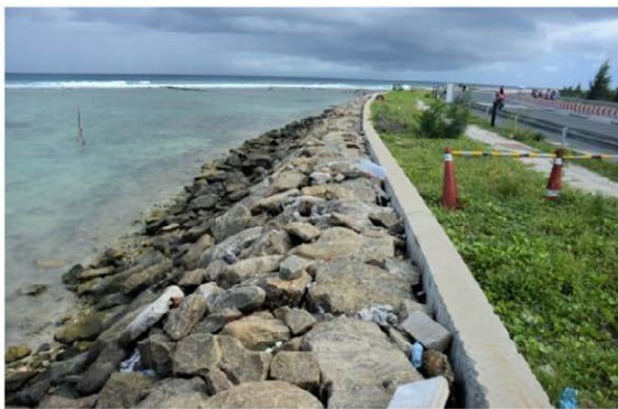
East seawall facing the open sea (the armor stone: +3.0 m)
