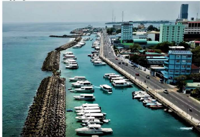
Detached breakwaters (L) and south seawall with quay function (R)
