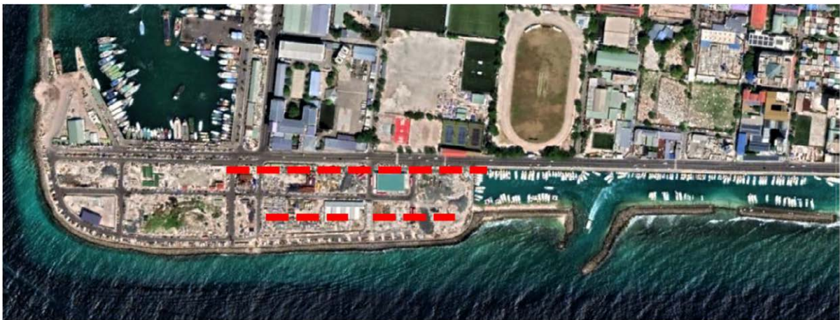
The red line is the seawall constructed by the ODA project, and the layout has been changed for the new shipping channel and harbor reclamation.
