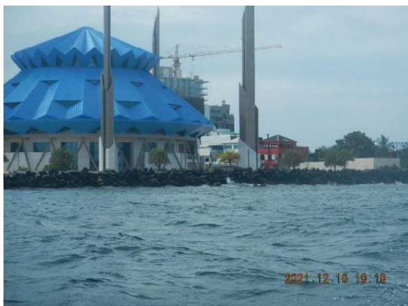
Figure2-1.1 Japanese seawall on the north side of the artificial beach on the east coast of Male' Island, 10 December 2021
