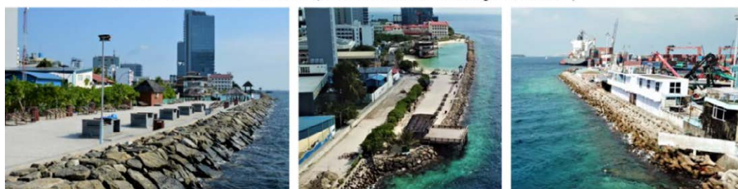
Large stones were used instead of tetrapods.
