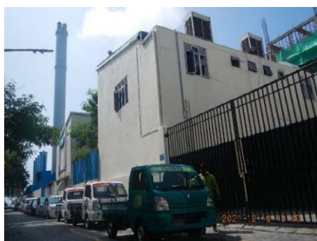
Figure 3-3.1 Desalination plant at MWSC
