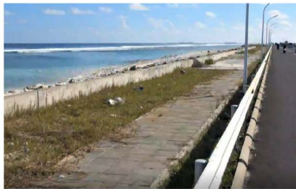
Pedestrian walkway between seawall and roadway.
