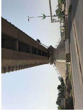
From the road surface to the bottom of the girder : 6.0m
