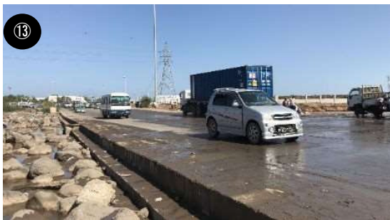
Ford structure that is flooded and cannot be used by traffic when rain falls.
