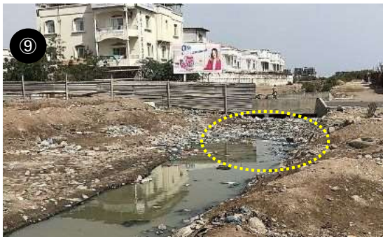
Ford structure that is flooded and cannot be used by traffic when rain falls.
