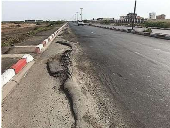
Road Condition in Djibouti City (Pavement Damage)
