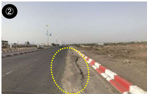
The width of the road is reduced due to rutting on the shoulder.
