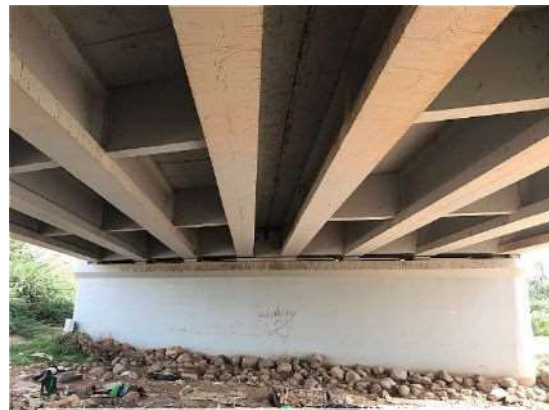
Condition under the girder of the Italy Bridge
