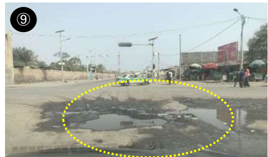
Pavement is deteriorating significantly.
