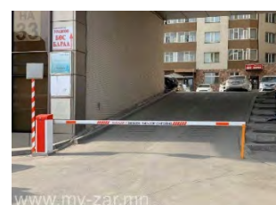
Installation of Retractable Gates
