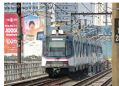
Elevated Railway with Tram type Rolling Stock
