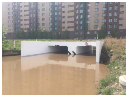
Source: https://gogo.mn/r/v5l0l Bayanmongol underpass
