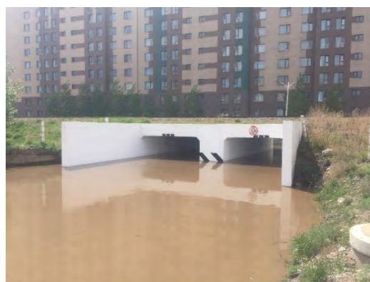
Source: https://gogo.mn/r/v5l0l Bayanmongol underpass
