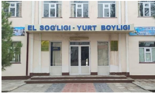
Entrance, Karmana District Central Hospital
