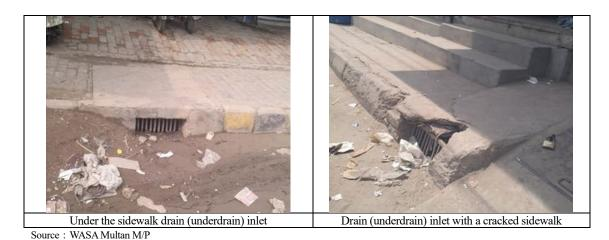
Figure 3.4-4 Roadside Drains
