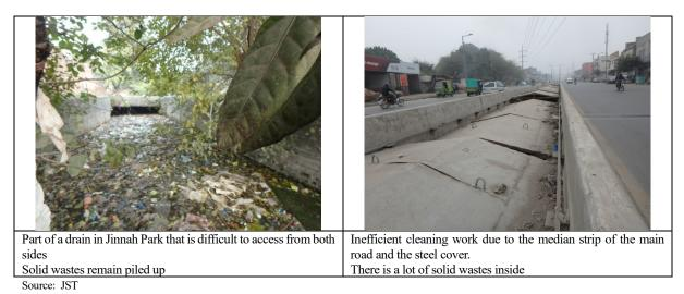
Figure 6.3-9 Drains Having Difficulty of Cleaning Work
