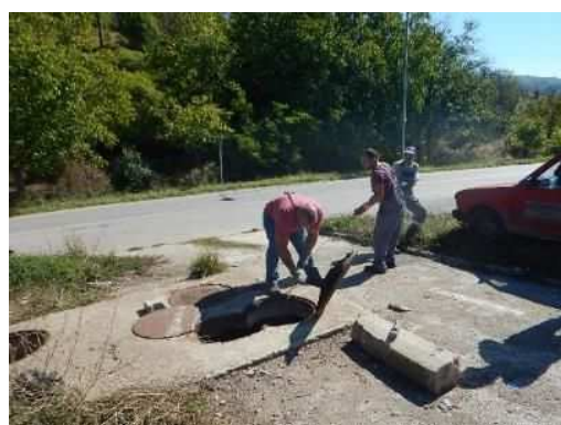
Pulling out a clogged pump.
