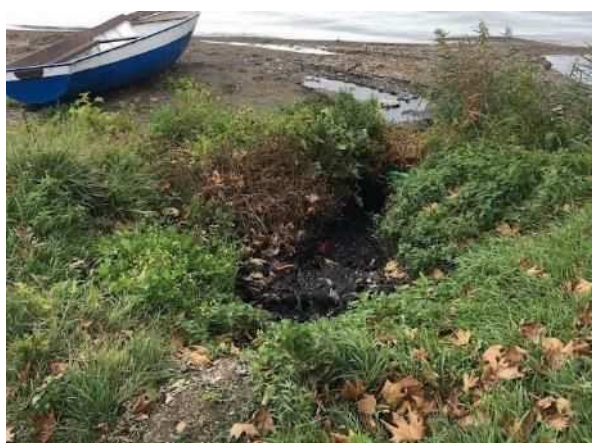
Discharge Point 2 (Dry weather)
