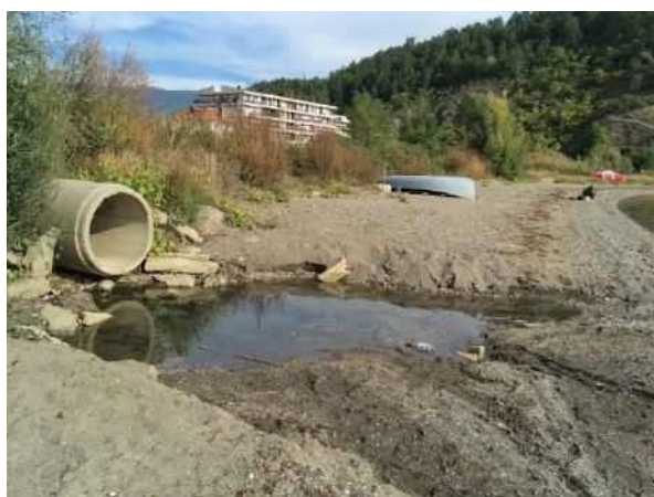
Discharge Point 1 (Dry weather)
