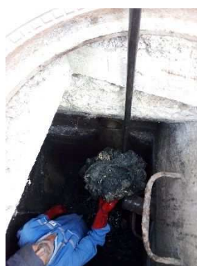
Cleaning sediment in a manhole by human power
