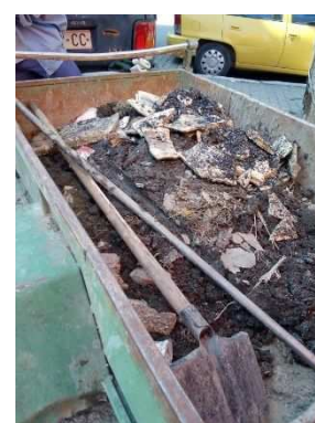
Sediment collected from inside sewer
