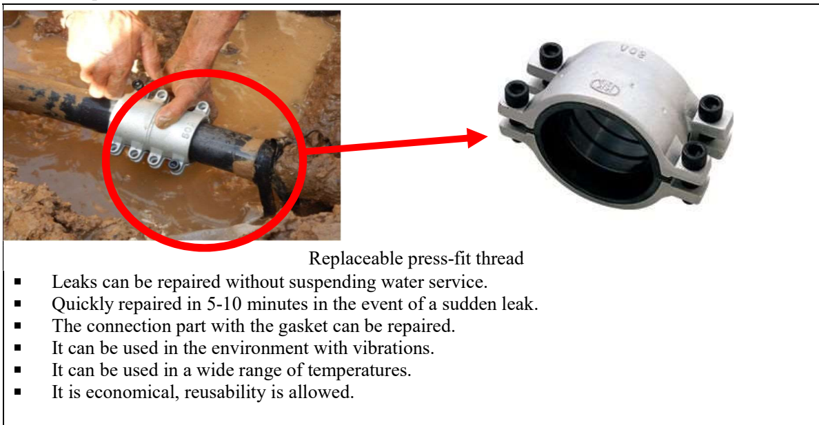
Figure 5-3-2 Repairing Leaks with Pressure Clamp
