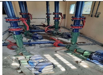
Chlorine dosing device
