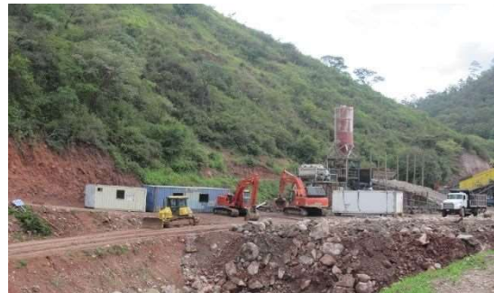
Temporary office for construction
