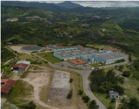
Photo 5 Aerial View of La Concepción Water Treatment Plant
