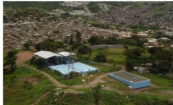
Photo 8 Miraflores Water Treatment Plant
