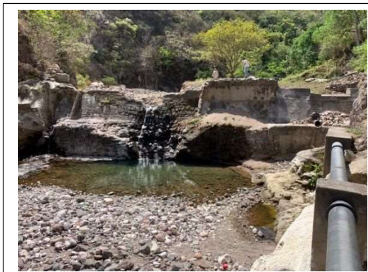
Intake work (front view)
