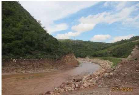
Spillway construction site (①).
