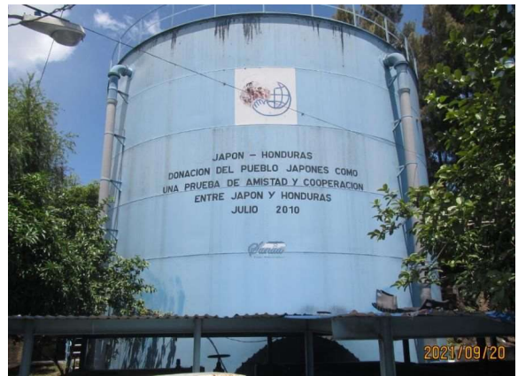
Photo 10 Olimpo 1 Distribution Tank
