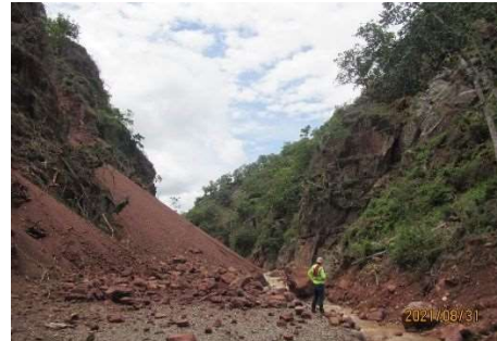
Dam construction site (②).
