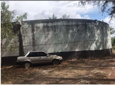
Photo 11 Los Filtros Distribution Tank
