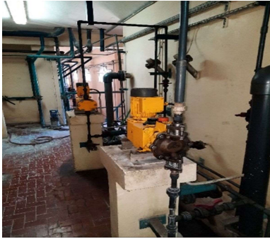
Activated carbon dosing pump
