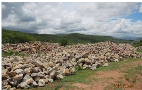
Water treatment plant construction site (③).
