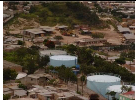
Photo 12 Olimpo 2 Distribution Tanks
