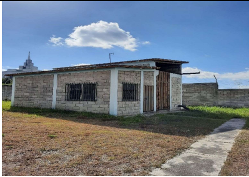
1. Pumping Station No.4 Roble Oeste VI (the most recent one)
