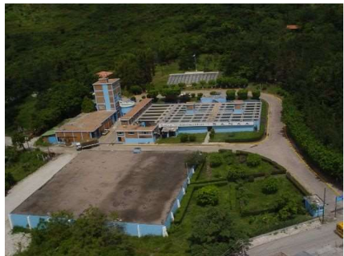
Photo 6 Los Laureles Water Treatment Plant
