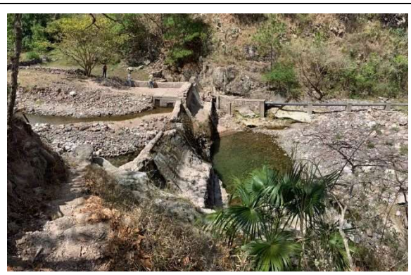
Intake work (side view)
