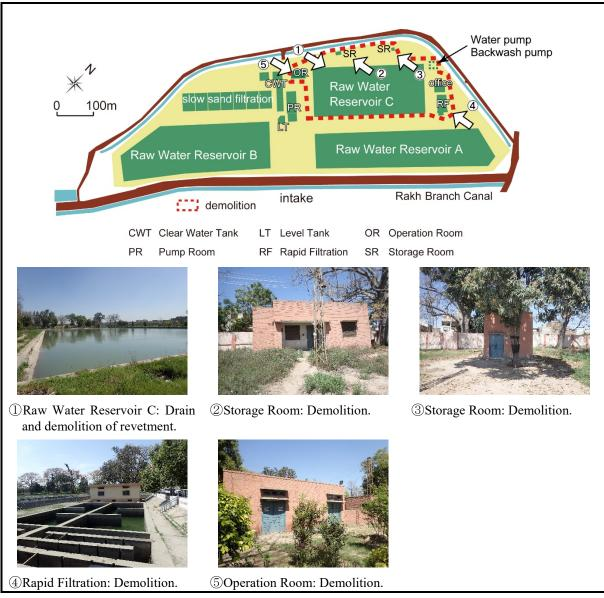
Figure 2-38 Dismantling of existing facilities at Old JK WTP
