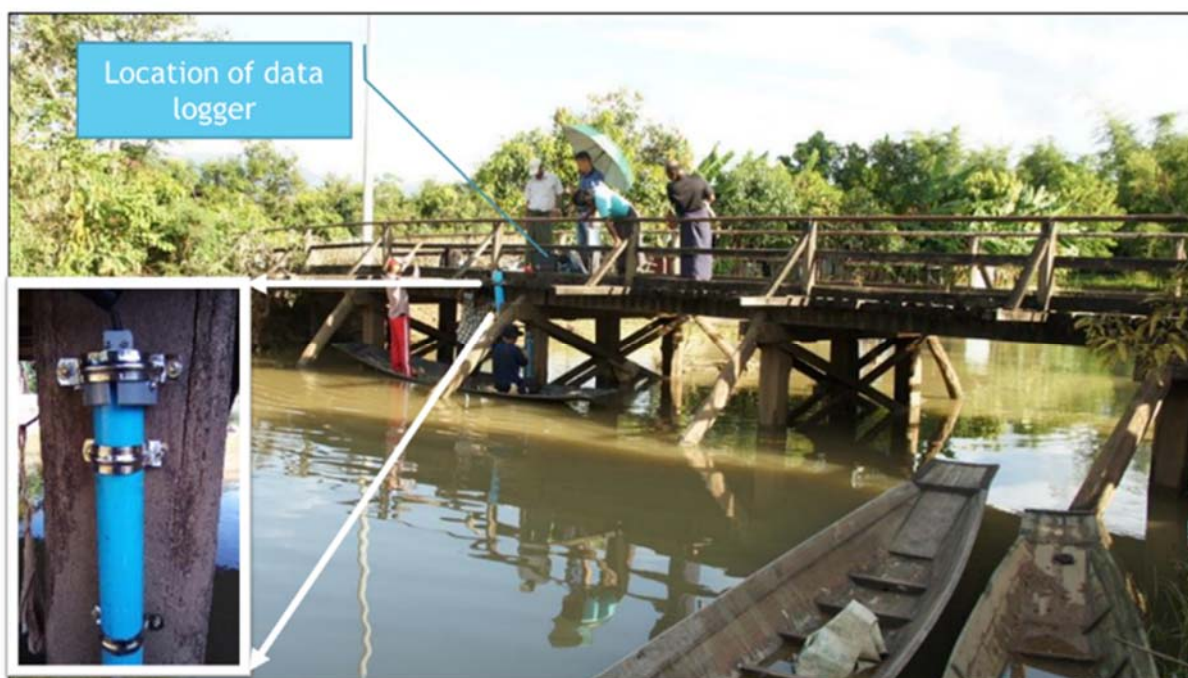
Fig5 Structure for water level monitoring (in case of Nam Lat river)
