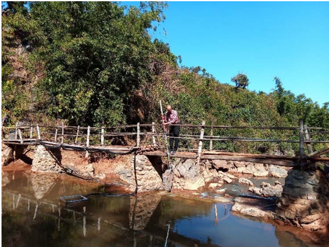
Fig12 Measurement of water flow velocity from bridge.
