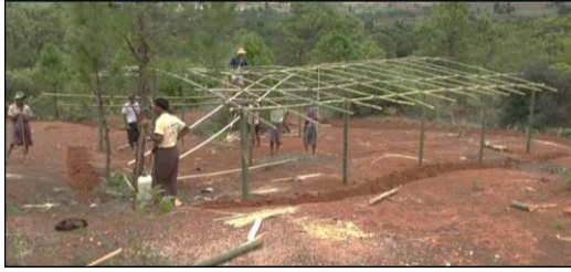
← Frame of temporary yard
