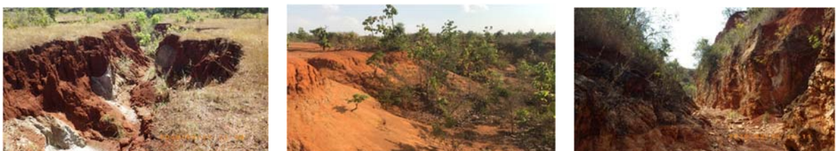
Figure 3 Example of gully erosion around Inle Lake area
