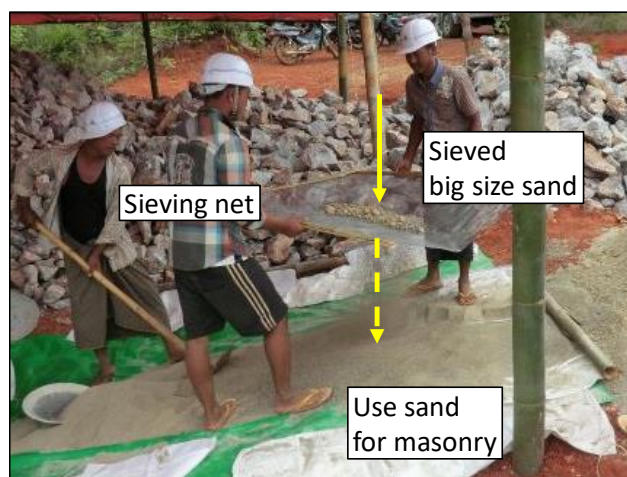
Figure 3.8-1 Sieving of Sand (Kon Ni Construction 2019)
