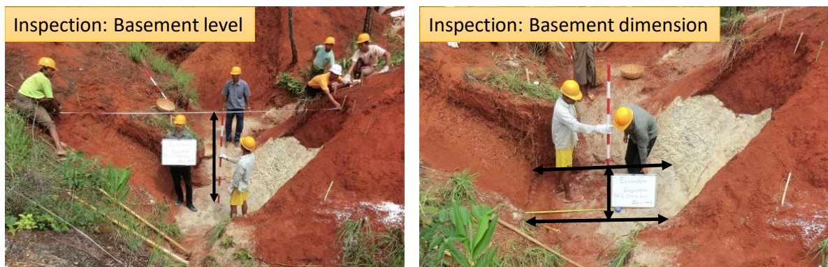
Figure 3.8-2 Inspection of Check Dam Excavation (Kon Ni Construction 2019)
