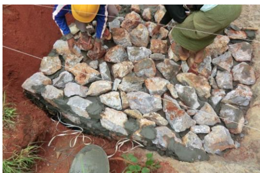
Figure 3.7-3 Masonry Work (Check Dam)
