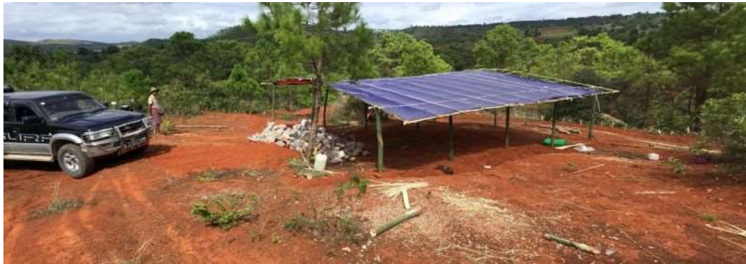
Setting of Temporary Yard
