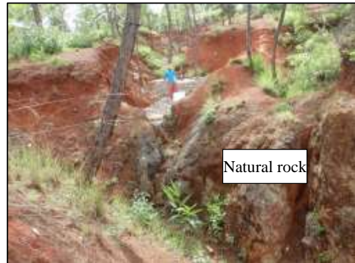
Overview from lower side
