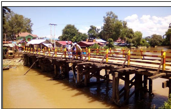
Water Level Gauge at the Bridge over Upper Balu
