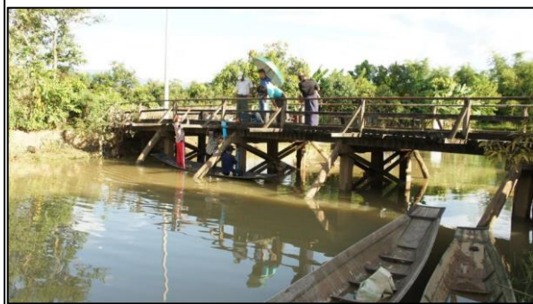
Water Level Gauge at the Bridge over Namlet
