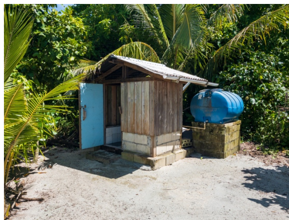
Toilet facilities on a remote island (Kayangel State)
