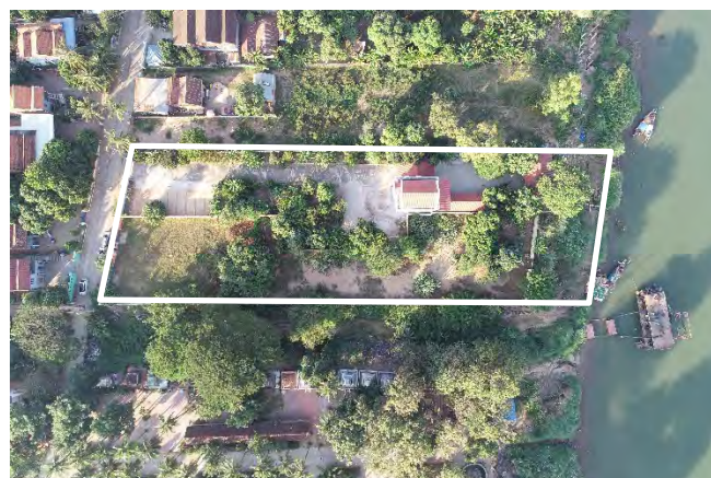
Figure 6.2.2 Appearance of candidate site for Raw Water Intake Facility (Bakheng Phase III)
