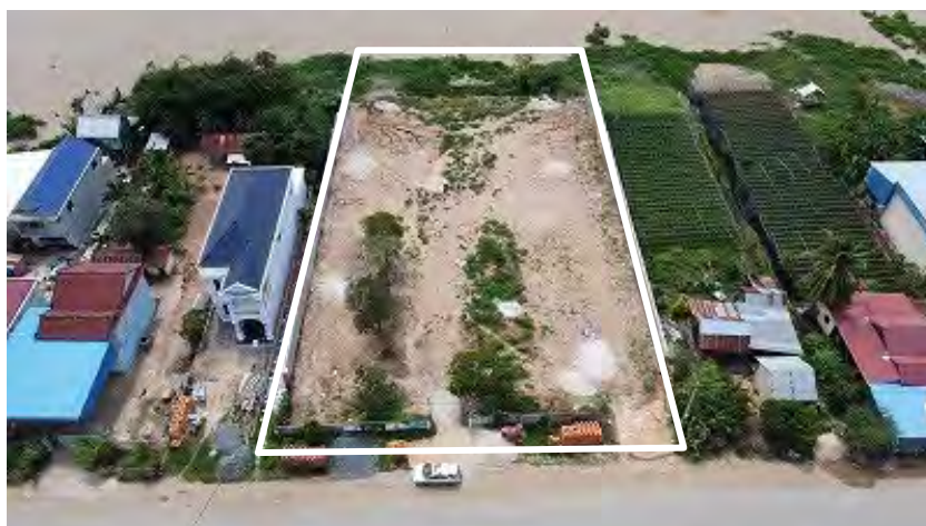
Figure 6.2.9 Appearance of Candidate Site for Raw Water Intake Facility of New Airport City (Option 1)
