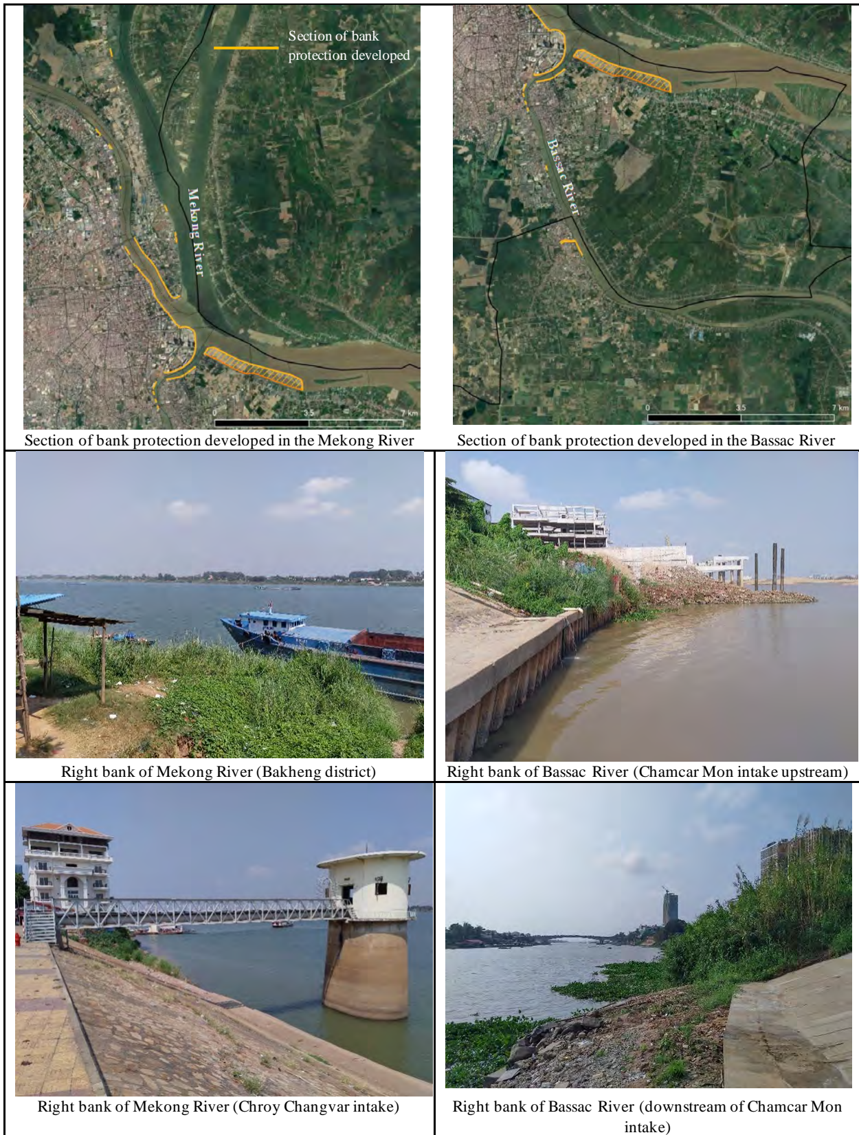
Figure 5.2.7 Riverbank erosion and revetment development in the Mekong and Bassac rivers Source: JICA Study Team based on MOWRAM data (2021)
