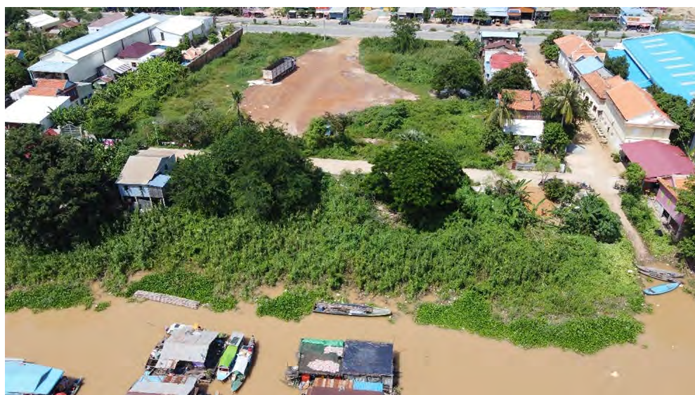
Figure 6.2.5 Appearance of Candidate Site for Intake Facility (Ta Mouk)
