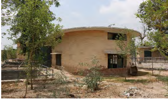
Disposal station D 2 Pump Room 1 (Old)
