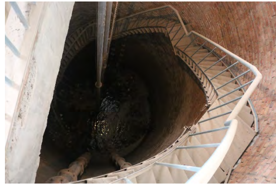
SUMBERSIBLE PUMP ROOM
