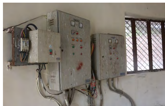
PUMP CONTROL PANEL
