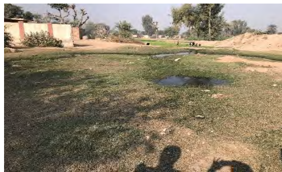
Leak point of Forced main on the site
