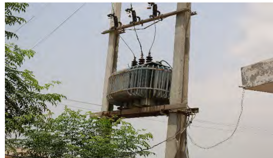
Pole-Mounted Transformer
