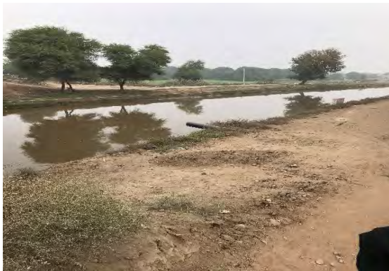
DISCHARGE TO CANAL
