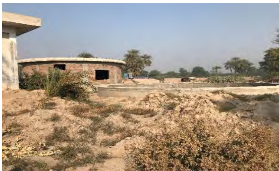
New No.2 pump facility under construction
