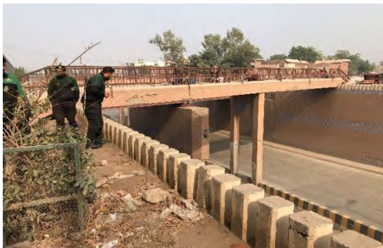
Under pass for drainage
