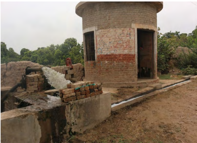
Pump discharge channel to farmland & Accompanying room
