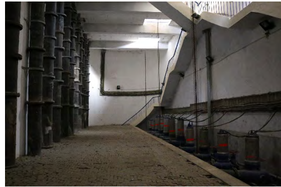
DRY-PIT TYPE SUBMERSIBLE PUMPS
