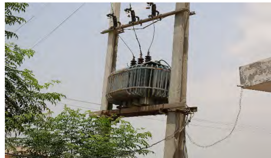
Pole-Mounted Transformer
