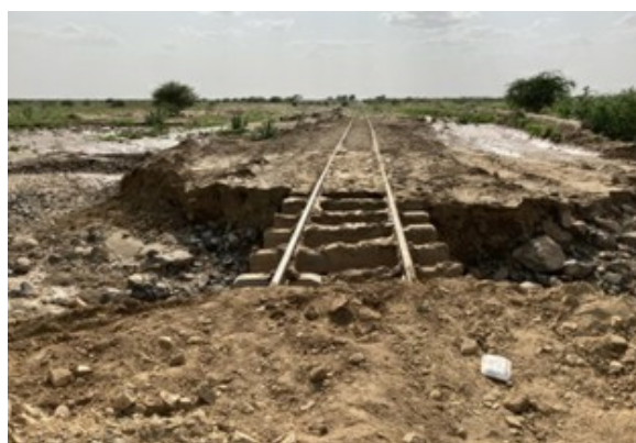
Figure 2-4-19 Flood Damage during the Rainy Season
