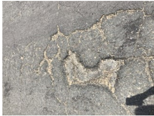
Road surface condition of Atbara-Haya road (Road pavement that needs to be repaired)
