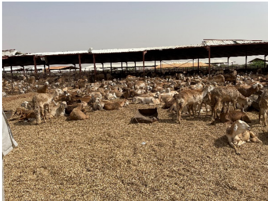
Quarantine Station at Khartoum State needs rehabilitation of roof, fence, etc.
