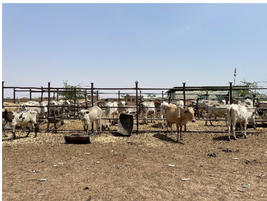
Livestock market at White Nile State needs rehabilitation of roof, water supply, etc.
