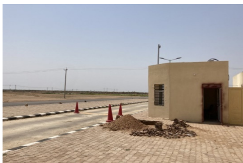
Equipment installation location: The target vehicle is weighed on the side lane (the left back is the main lane)
