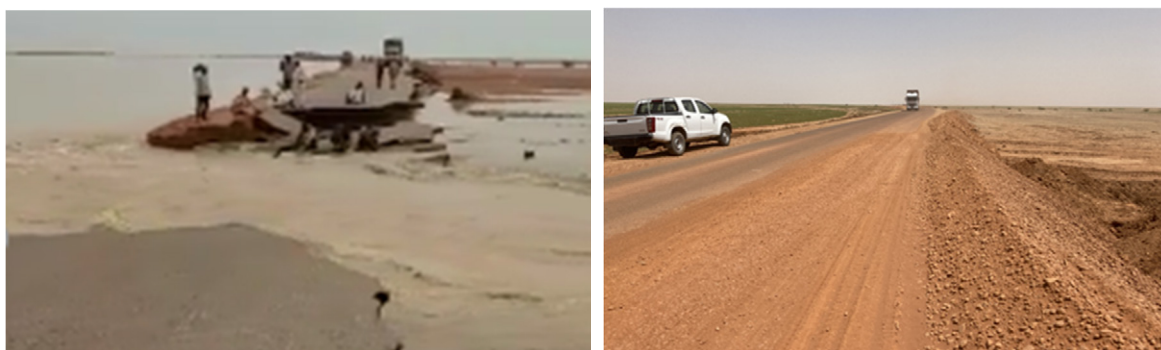
Figure 2-4-10 The Section Where Pavement and Embankment Collapsed Due to Flooding and the Road after Emergency Repair of the Same Section (between Atbara and Suakin)
