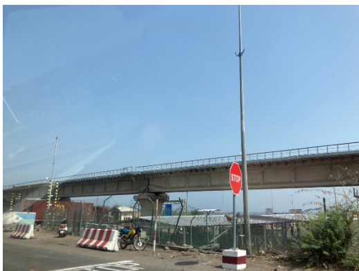
Djibouti-Addis Ababa Railway
