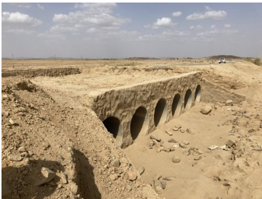
New Box Culvert on Atbara-Haya Road
