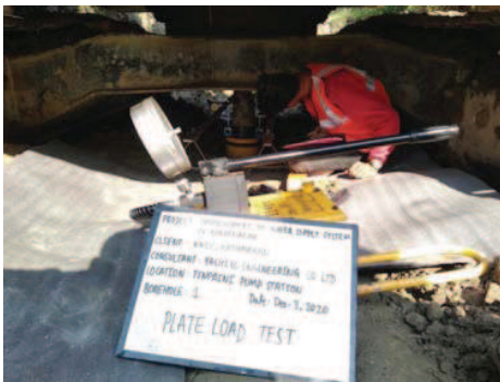
Photo-5: Recording field test data
