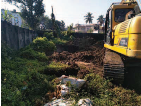
Photo-2: Excavating the trial pit at the depth of 1.5m
