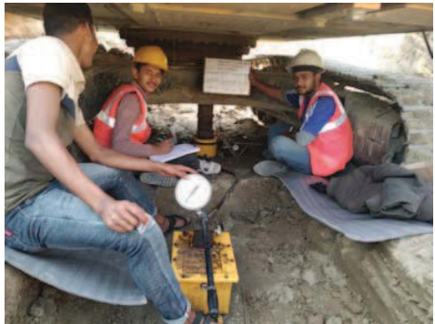
Photo-7: Providing Hydraulic loading
