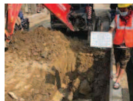
Fig. Site Condition of Trial Pit Location
