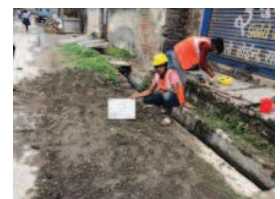
Fig. Test Pit After Backfill
