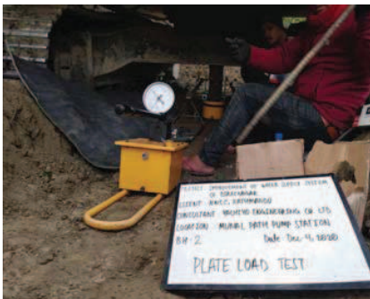
Photo-5: Recording field test data
