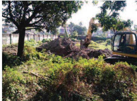
Photo-8: Excavator at site
