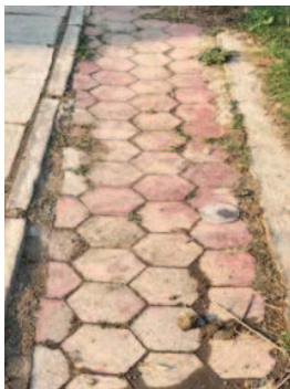
Fig. Trial Pit location Before Excavation
