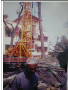
Photo No.1 : Tubewell Drill by Direct Rotary method.
