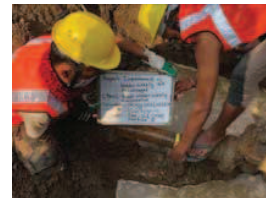
Fig. Helper Measuring the External Diameter of Water Supply Pipe
