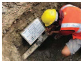
Fig. Helper Measuring External Dia. Of Pipe
