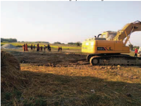
Photo-8: Excavator at site
