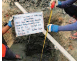
Fig. Helper Measuring Depth of Water Supply Pipe from Surface
