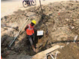
Fig. Helper Measuring Pipe Depth From Surface
