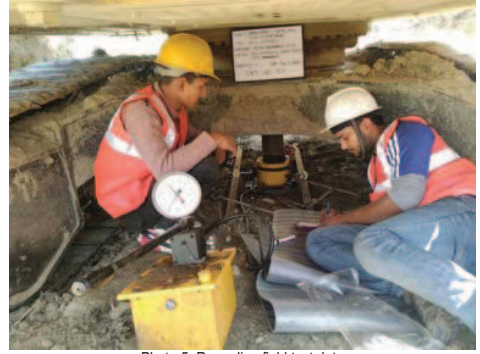
Photo-5: Recording field test data
