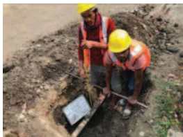
Fig. Helper Measuring Pipe Depth From Surface
