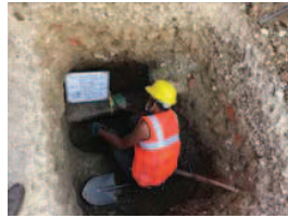
Fig. Helper Measuring External Dia. of Pipe
