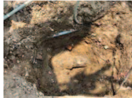
Fig. Condition of DI Pipe after Excavation
