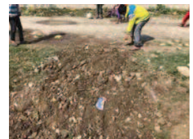
Fig. Test Pit After Backfill
