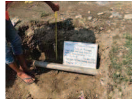
Fig. Helper Measuring Pipe Depth From Surface
