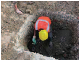
Fig. Helper Compacting During Backfill
