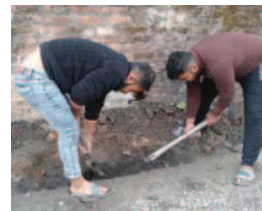
Fig. Helper Excavating Test Pit
