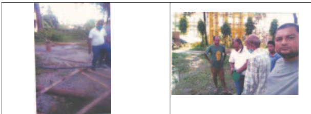
Photo No.: 13 Compressor pipe lowering for well development by compressor.
