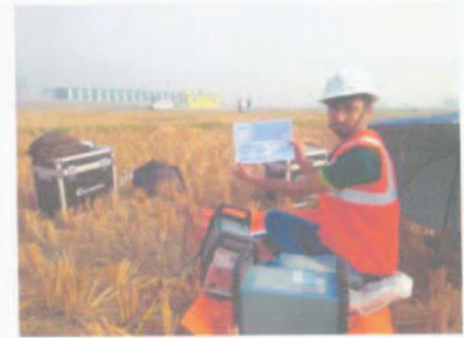
Cable Layout and Data acquisition of VES-9 (NWSC- 1)
