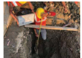
Fig. Helper Measuring Depth of Water Supply Pipe from Surface
