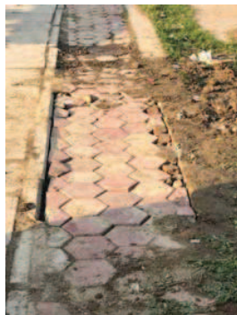
Fig. Trial Pit location After Excavation
