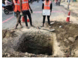
Fig. Test Pit After Excavation
