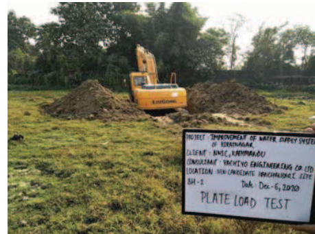
Photo-1: Trial Pit Excavation for PLT test
