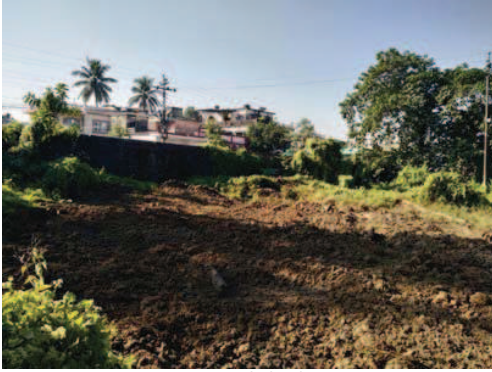
Photo-1: Preparing Surface for PLT test
