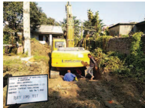
Photo-7: Providing Hydraulic loading
