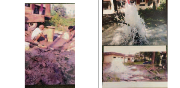
Photo No 5: Bore hole top sealing with 1m concrete.
