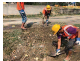
Fig. Test Pit Being Backfilled
