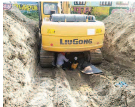
Photo-7: Providing Hydraulic loading
