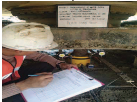
Photo-6: Recording field test data
