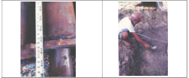
Photo No. 9: Joining of MS pipe by welding.
