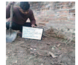
Fig. Test Pit Location After Backfill
