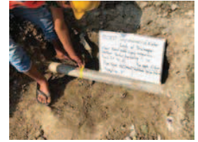
Fig. Helper Measuring External Dia. Of Pipe
