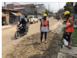
Fig. Test Pit After Backfill
