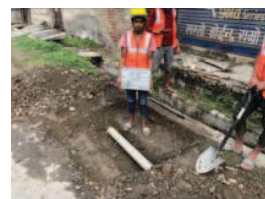
Fig. Test Pit After Excavation
