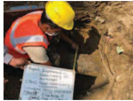
Fig. Helper Measuring External Dia. Of Pipe
