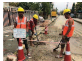
Fig. Site Condition of Trial Pit location before Excavation
