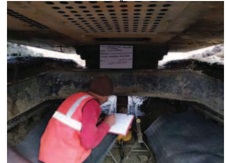
Photo-6: Recording field test data
