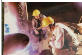
Photo No.3: Inspection of casing welding, 14 March 2020.
