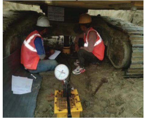
Photo-6: Recording field test data
