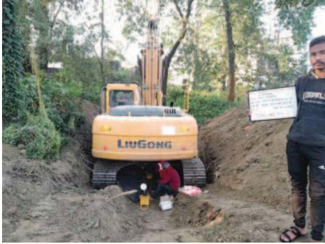
Photo-1: Trial Pit Excavation for PLT test
