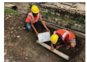
Fig. Helper Measuring External Dia. Of Pipe
