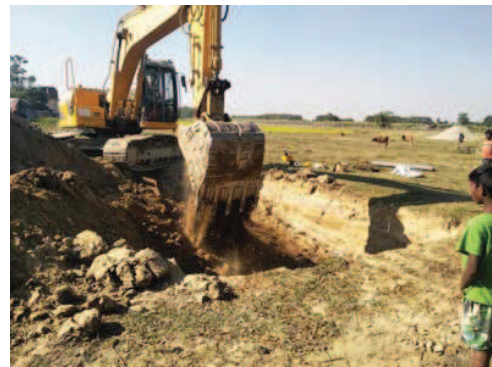
Photo-1: Trial Pit Excavation for PLT test
