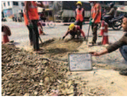
Fig. Site Condition Before Excavation of Test Pit
