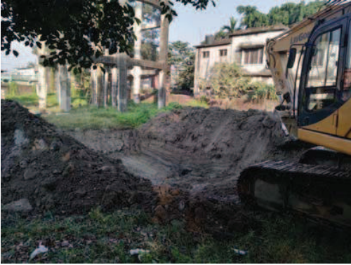
Photo-1: Trial Pit Excavation for PLT test
