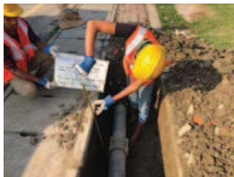
Fig. Measuring Pipe Depth From Surface
