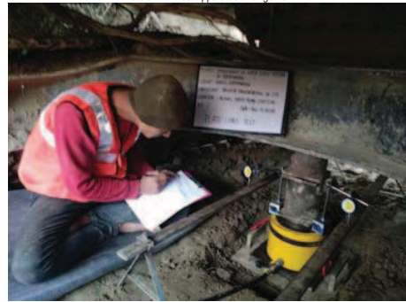
Photo-4: Recording field test data
