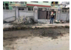
Fig. Test Pit Location After Backfill
