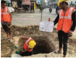
Fig. Helper Measuring Pipe Depth From Surface
