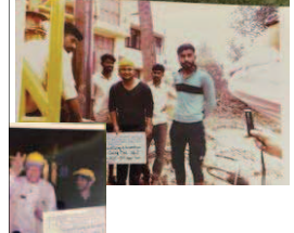
Photo No.4: Installation of Casing and screen, 14 March 2020
