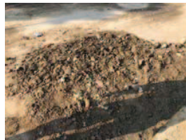
Fig. Test Pit After Backfill
