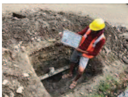
Fig. Test Pit After Excavation
