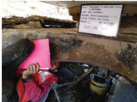
Photo-6: Recording field test data
