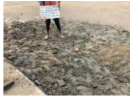
Fig. Test Pit Location After Backfill
