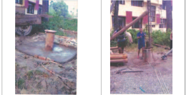
Photo No.: 11 Completion of Bore hole top concreting.
