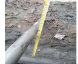
Fig. Helper Measuring Depth of Water Supply Pipe from Surface
