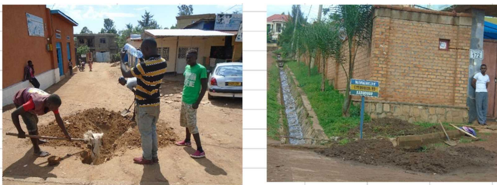
Test excavation at sites
