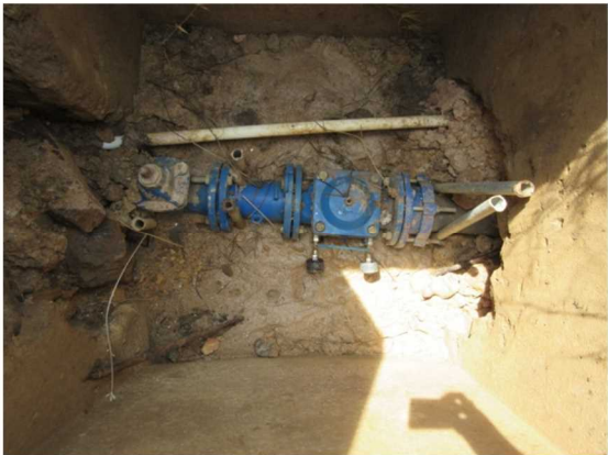
Standard installation and composition of PRV of WASAC
