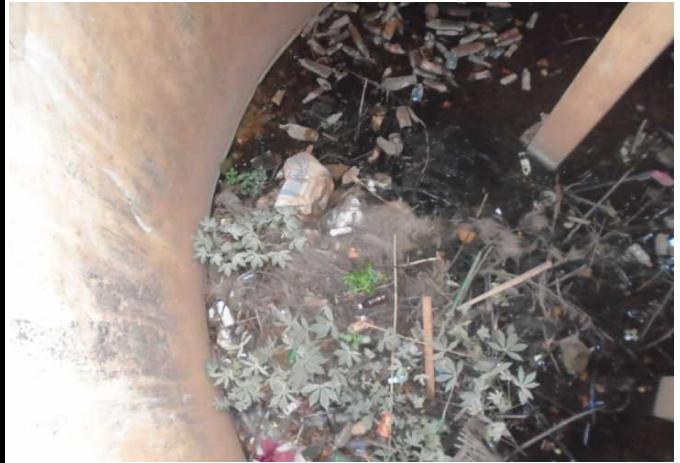
Inside of abandoned Reservoir
