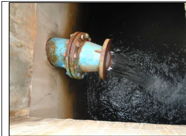
Floater valve needed
