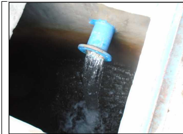
Floater valve needed
