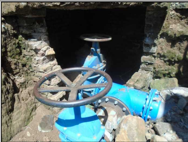
Rehabilitation of inlet manhole
