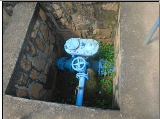
Covering of manhole
