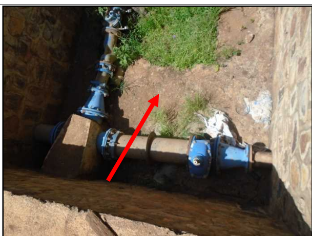
Manhoke bottom concreting works and covering
