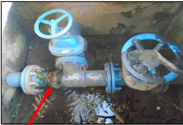
Leaking Tee
