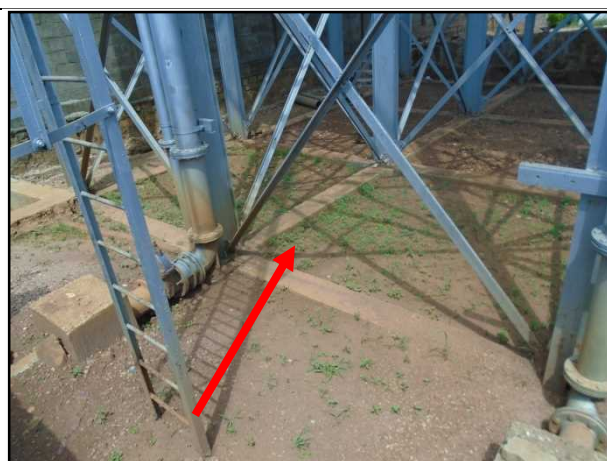
Bottom floor concreting for support protection
