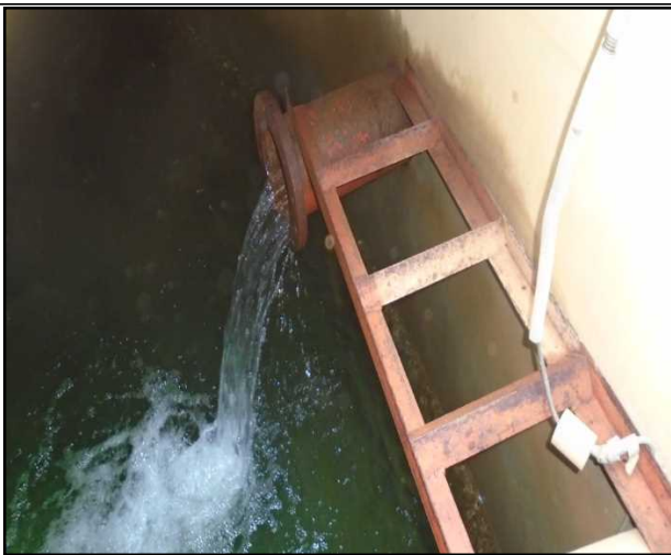
Floater Valve needed.
