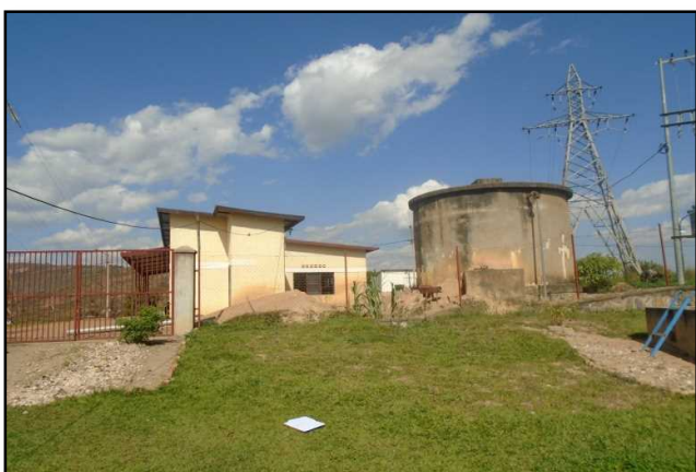
Support Reservoir located behind pump house. Capacity: 25m3
