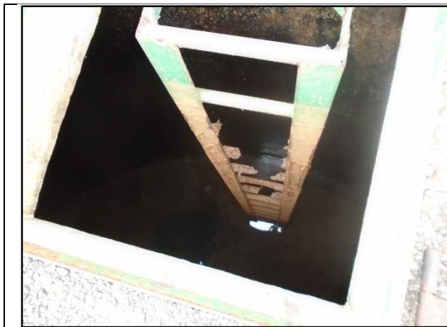
Floater valve needed
