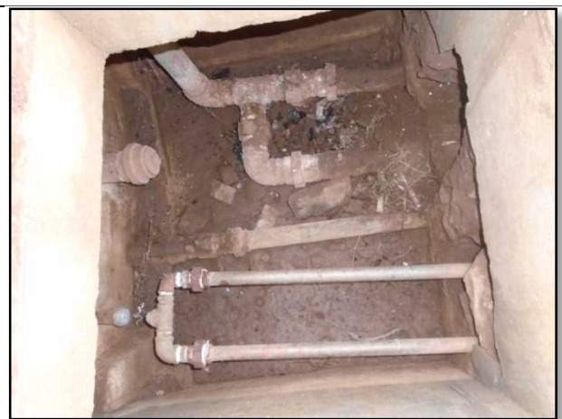
Reconnection and outlet accessories needed
