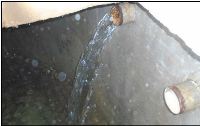
Floater valve needed
