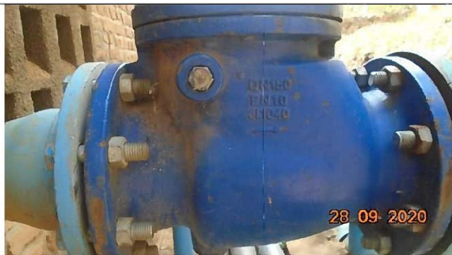
Replacement of non-functioning Check Valve
