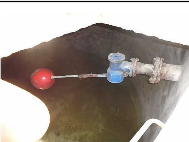
Inlet Pipe with Valve
