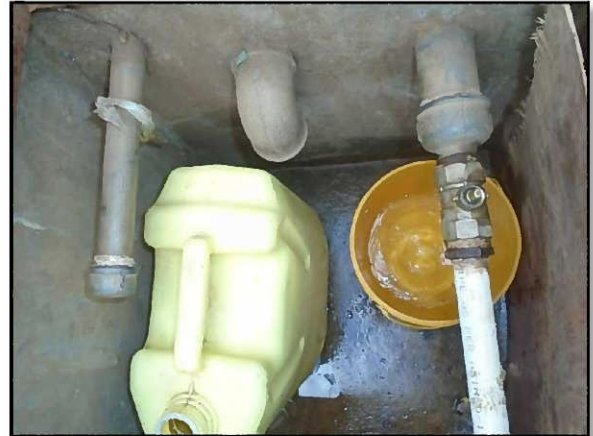
Replacement of outlet valve
