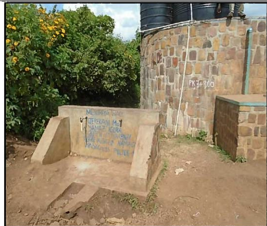
Reconnection to the existing Public Water Tap
