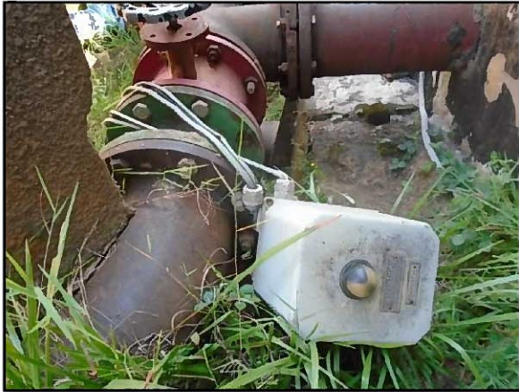
Defective Electrovalve
