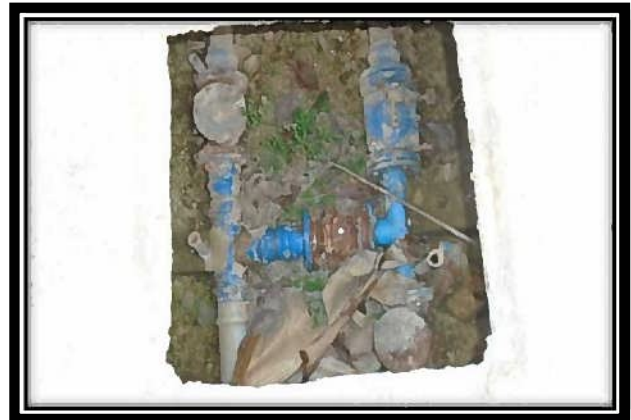
Outlet Pipe with Valve
