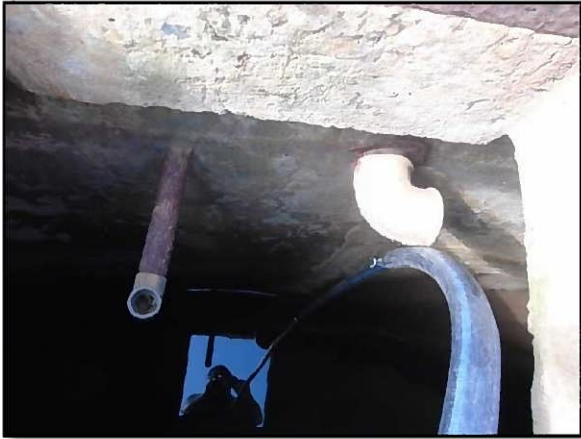
Floater valver needed
