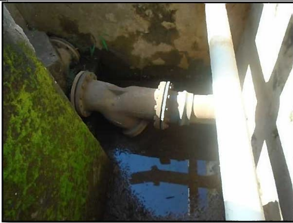
Rainwater drainage system needed.
