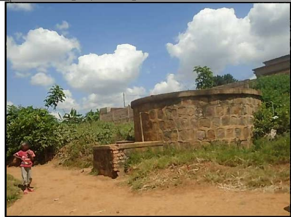
Reservoir in road dimension.
