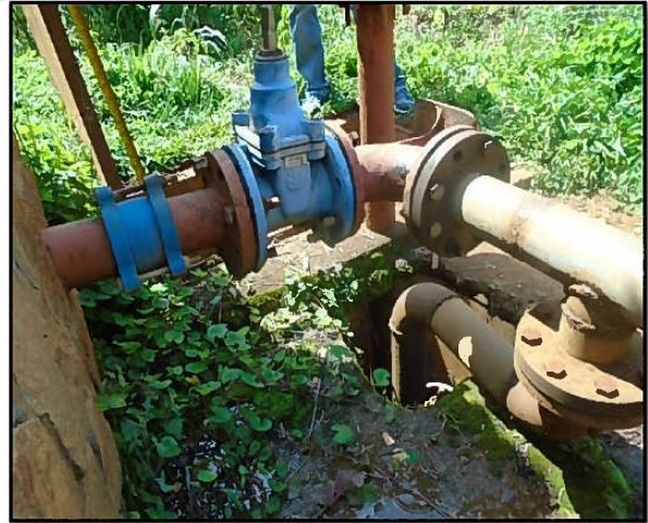
Wall leaks at the connection of the manhole
