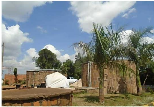
Inlet Pipe with Valve
