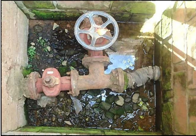
Outlet Collection Chamber DN80
