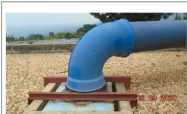
Floater on DN400 Pipe needed
