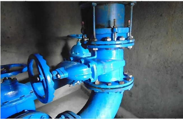
Inlet Pipe with Valve
