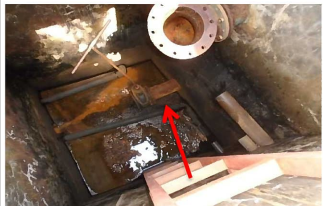
Outlet Pipe with Valve
