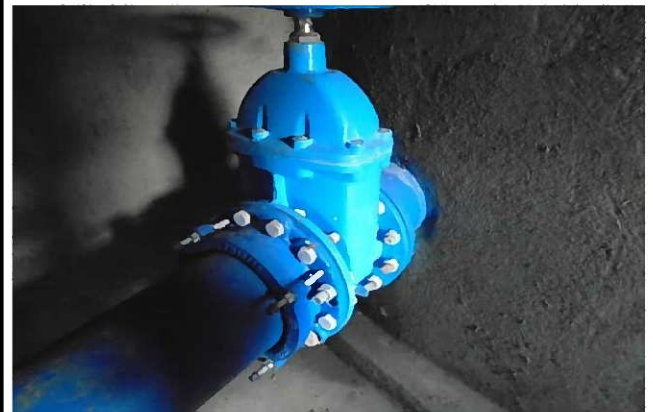
Outlet Pipe with Valve
