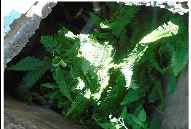
Outlet Pipe with Valve
