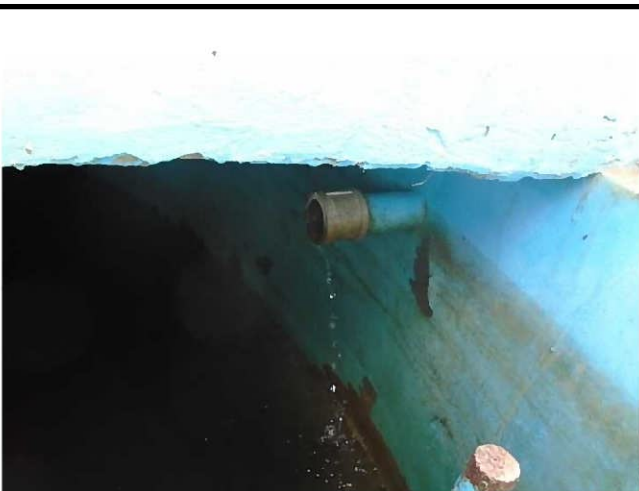
Inlet Pipe with Valve
