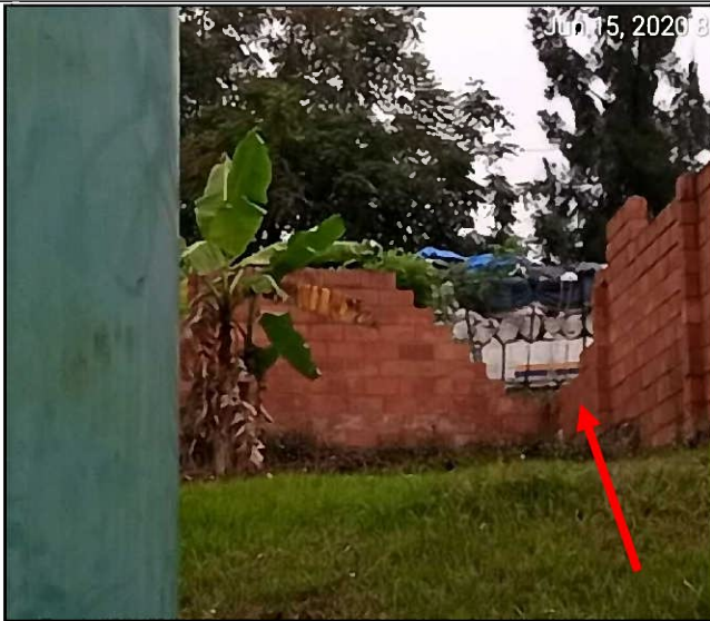
These fallen part of fence are being used by thieves and intruders
