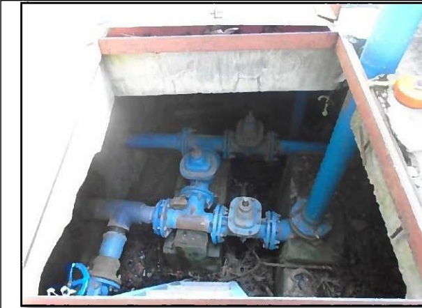
Manhole cover replacement
