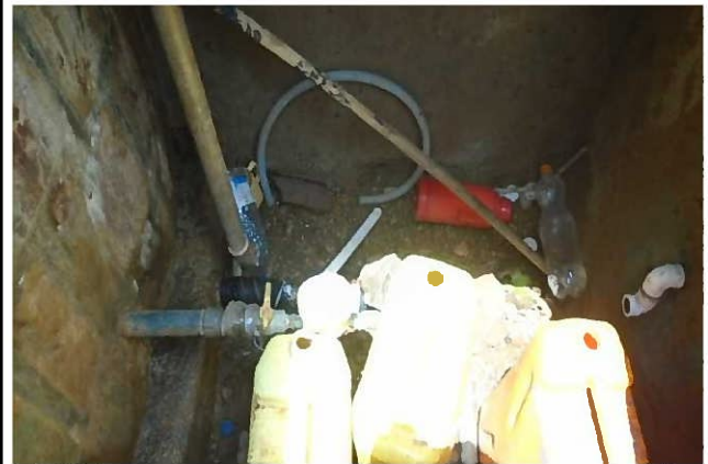
Outlet Pipe with Valve
