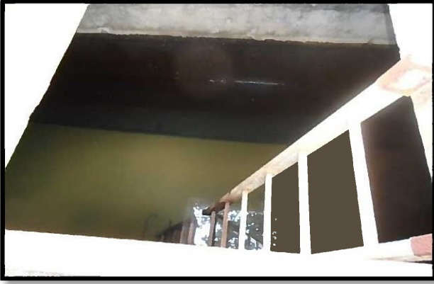
Inside of Manhole
