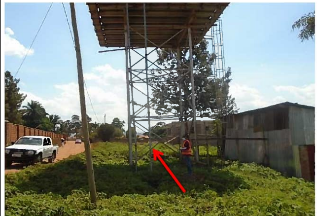
Outlet Pipe with Valve
