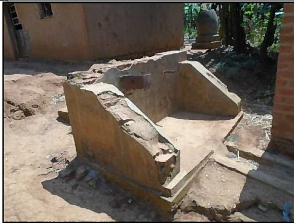
Rehabilitation of the nearby Water Tap will be necessary if reservoir is needed
