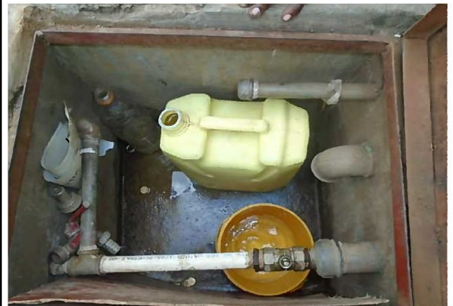
Outlet Pipe with Valve
