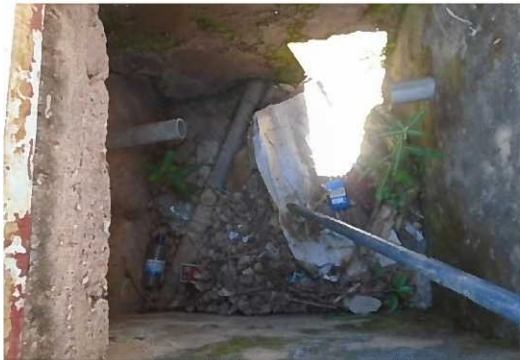
Inlet Pipe with Valve
