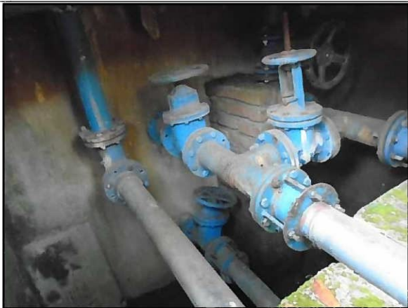
Replacement of all 4 valves
