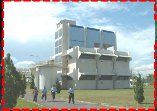
Somba Opu Water Treatment Plant (3300 l/s)
