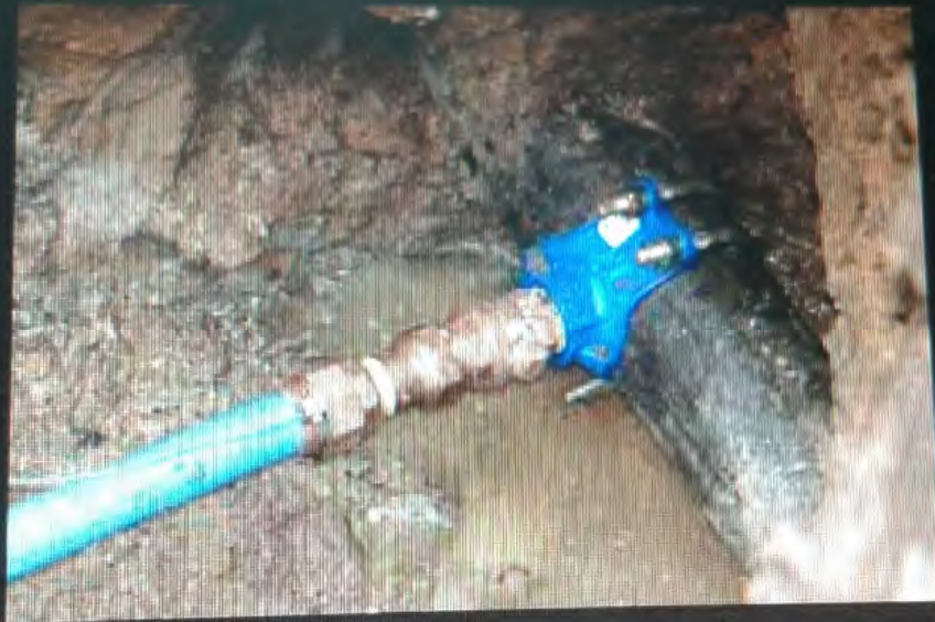
Screwed clamp, Valve, Union, socket, PE pipe
