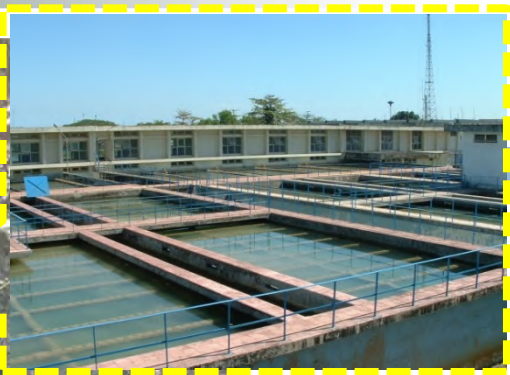
Panaikang Water Treatment Plant (1100 l/s)
