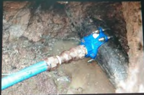
Screwed clamp, Valve, Union, socket, PE pipe
