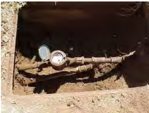
Examples of an illegal bypass around a meter—another form of theft and one of the causes of commercial losses.
