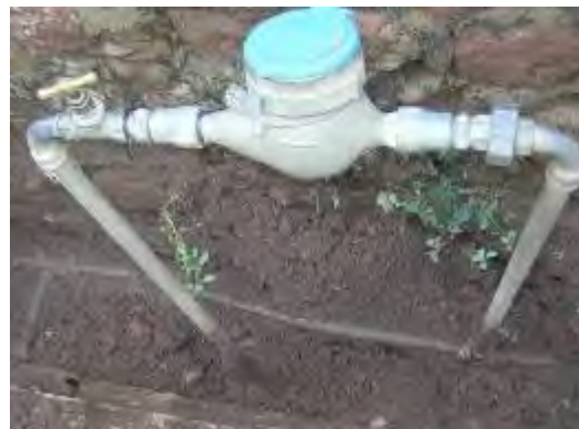
Examples of an illegal bypass around a meter—another form of theft and one of the causes of commercial losses.
