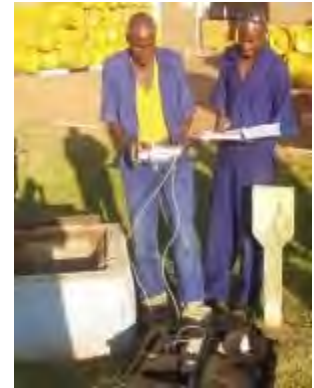
Field verification of the network data is crucial to understanding where water losses originate and setting NRW baseline level.
