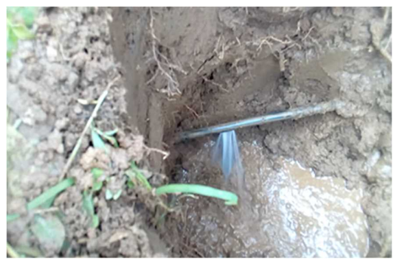
Underground Leakage
