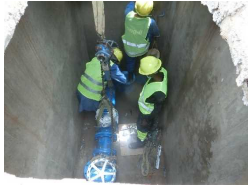
Installation of Flow Meter of Monitoring System
