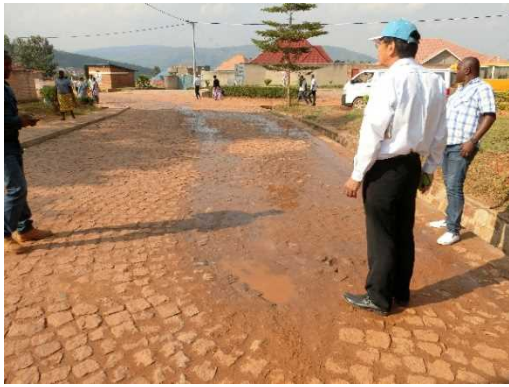
Surface Leakage
