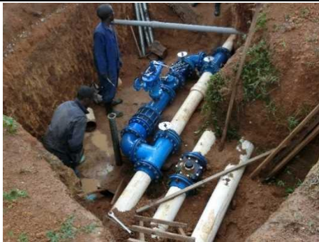
PRV Installation
