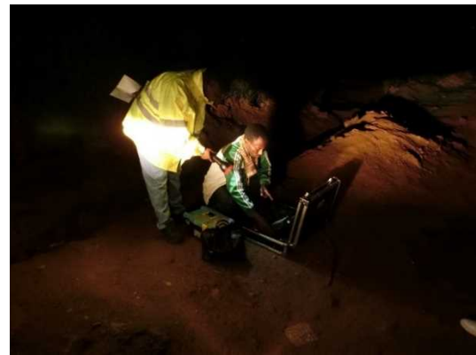
Minimum Nighttime Flow measurement
