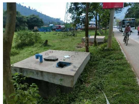
Manhole for Installation of Electromagnetic Flow meter
