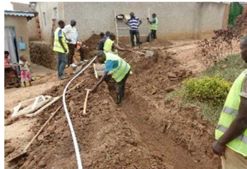
Replacement of Distribution Pipe
