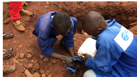
③ Clean the rubber of Saddle
