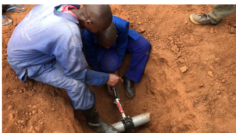
⑨ Close the gate valve and remove drilling
