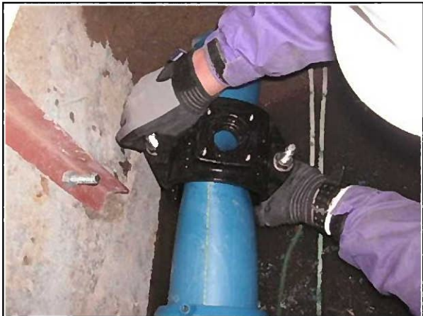
Reforming of flattened part
