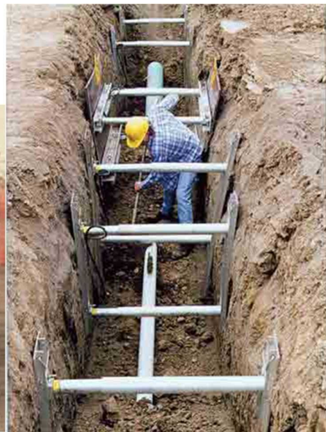
Fig.21 Soil Retaining Wall 2
