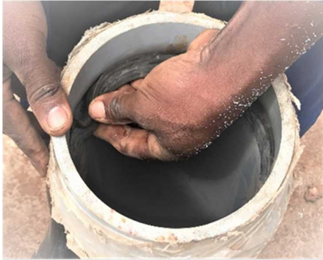
Fig.13 Setting a rubber ring
