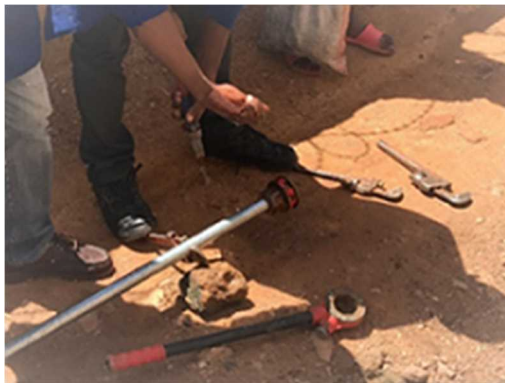
Fig.27 condition of screwing pipe
