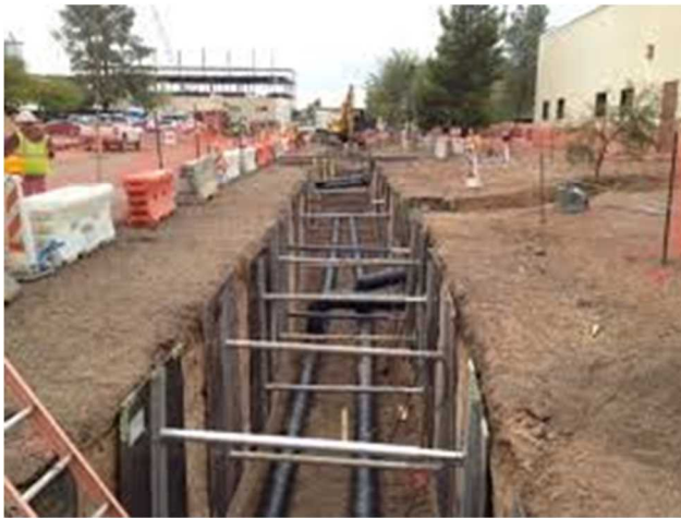
Fig.20 Soil Retaining Wall 1
