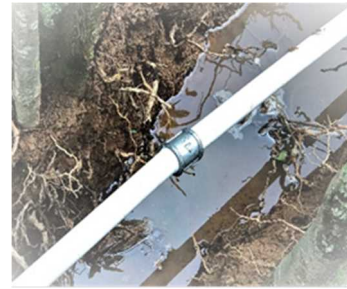
Fig.10 Coupling (screw)
