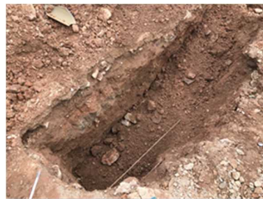
Fig.25 Pipe laying condition
