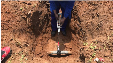
⑤ Fit the Drilling machine
