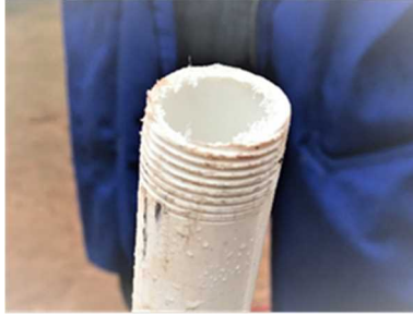
Fig.9 Screwing of uPVC
