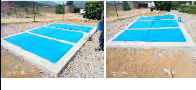
Top finishing after manhole covering and Application of paint photos
