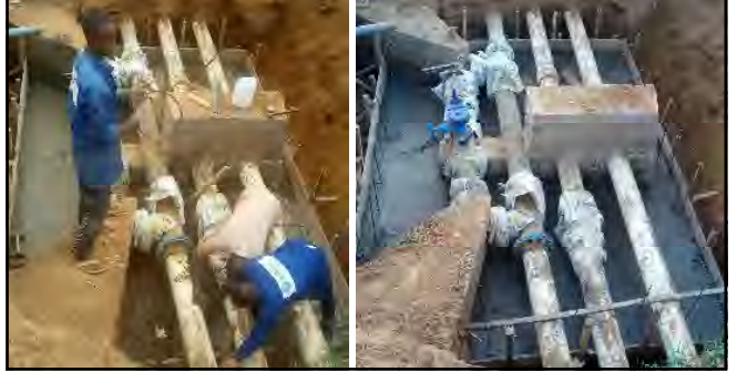
Slab concrete photos
