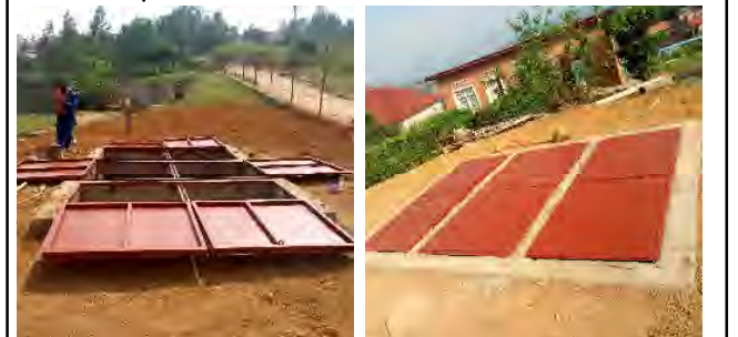
Manhole cover by welding metal tubes & metal sheet photos
