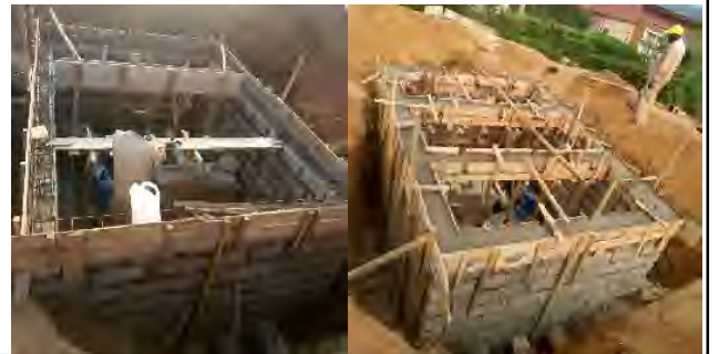
Steel bars, form work and Concrete for chaining & Beam
