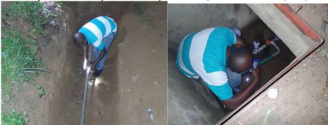
Installation of ultrasonic flow meter
