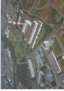
(Tsuzuki WtE incineration Plant)
