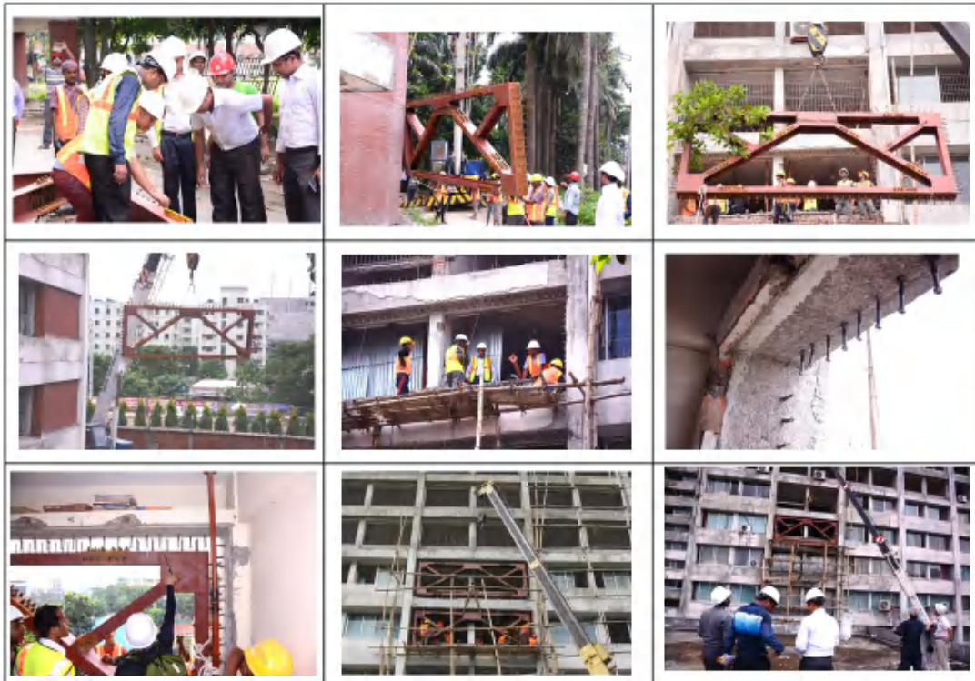
Steel Bracing Works at Radio Center in Agargaon
