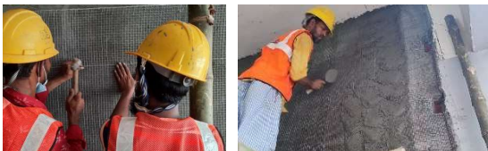
Test for Ferro-Cement Lamination on Masonry Infill
