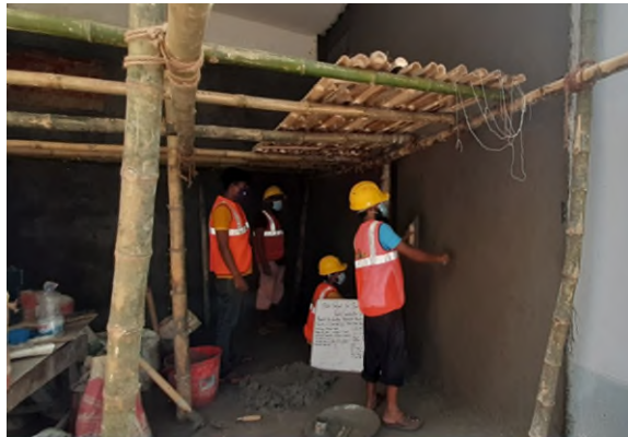
Ferrocement mortar work
