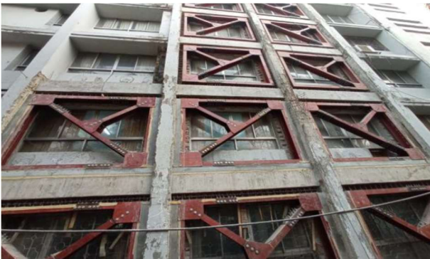
Retrofitting Work at BMD
