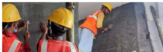
Test for Ferro-Cement Lamination on Masonry Infill (TSUIB: Technical Development to Upgrade Structural Integrity of Buildings in Densely Populated Urban Areas and Its Strategic Implementation towards Resilient Cities in Bangladesh”, and SATREPS: Science
