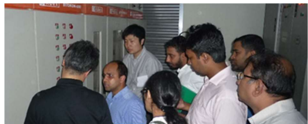
Observation and inspection of equipment
