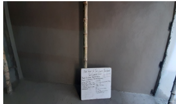
Ferrocement mortar work
