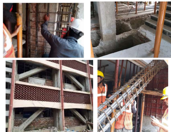
Retrofitting at PWD-HQ
