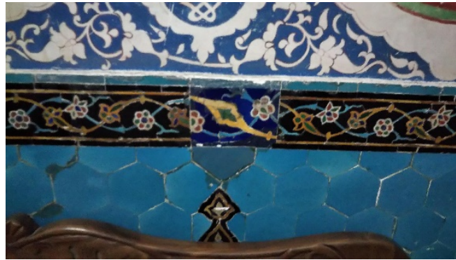
Figure 1.2: Inappropriate restoration at the Shah-i-Zinda
