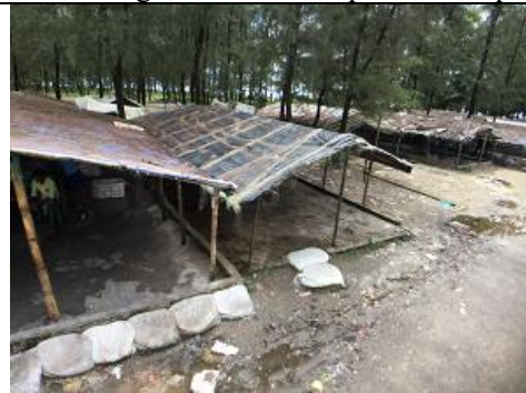
Shaplapur Landing Site (Shipping shed for landed fish along access road)
