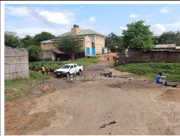
No.3 橋梁の現況
