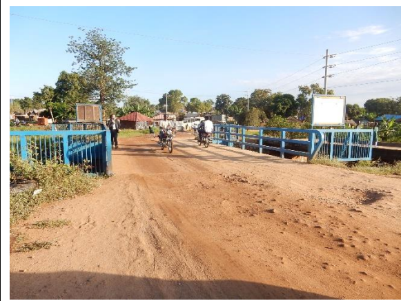
No.21 橋梁の現況
