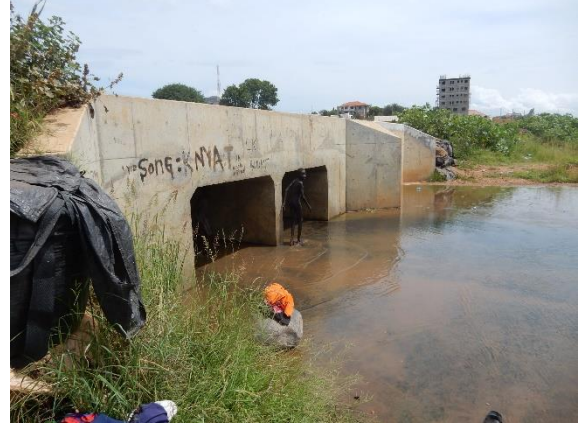
No.19 橋梁の現況
