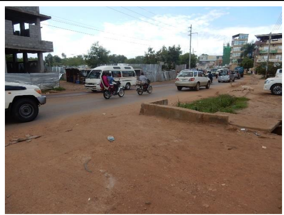
No.11 橋梁の現況
