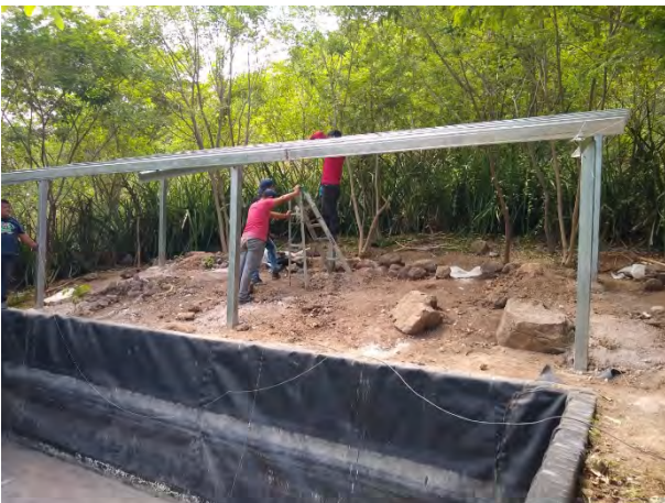
Photo 3: Las Perlas initiated remodeling of the reservoir with metallic materials for longer life in NPA Las Moritas on May 07 th (Las Moritas, San Miguel).
