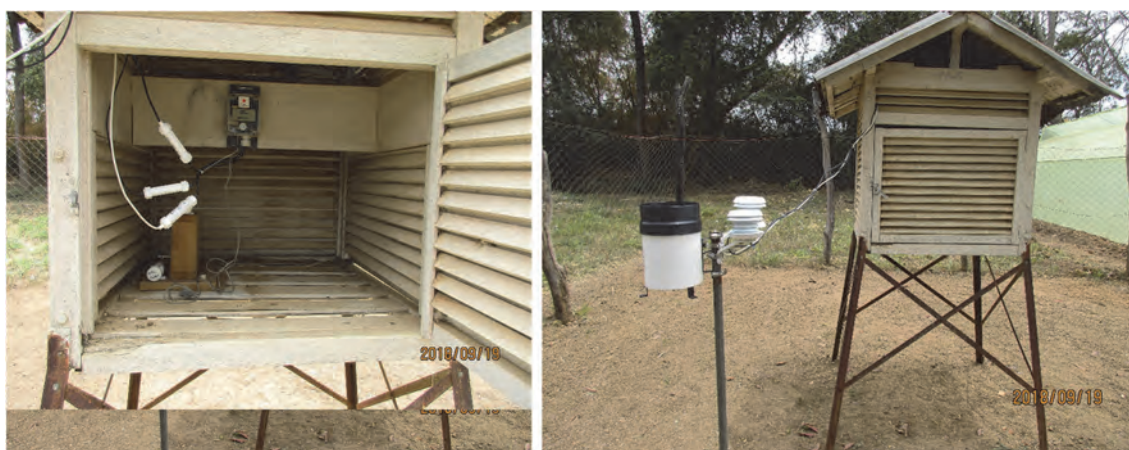
Photo 1 Equipment installation of weather station at Kitui Center
