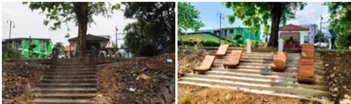
Figure 2.3.65 Zone 2 Before and After Improvement - 3
