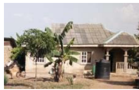
concrete in Berese
