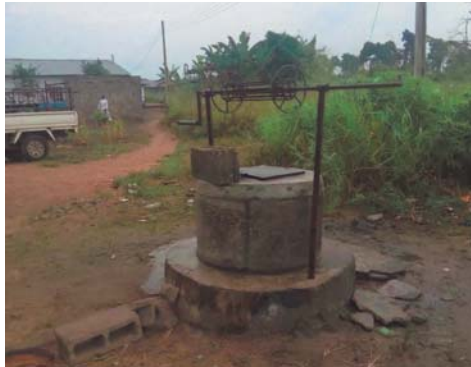
Plate 5.10: Community water well facility in Olorunsogo Community
