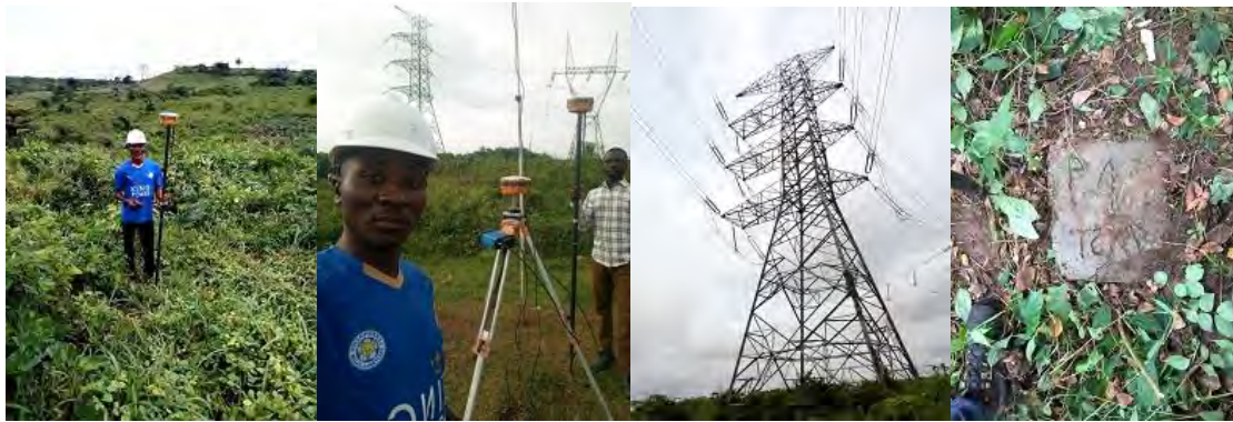
Figure 3: Topo Data Capturing, GPS set up, Tower and Boundary Point.
