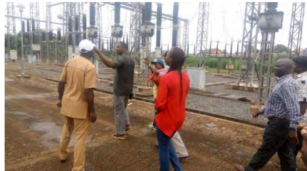
At Ikeja West Substation
