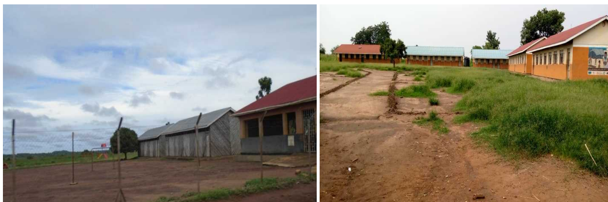
Figure 3-158: Most educational facilities like schools are built on public Land for example like at Adjumani in the pictures above.
