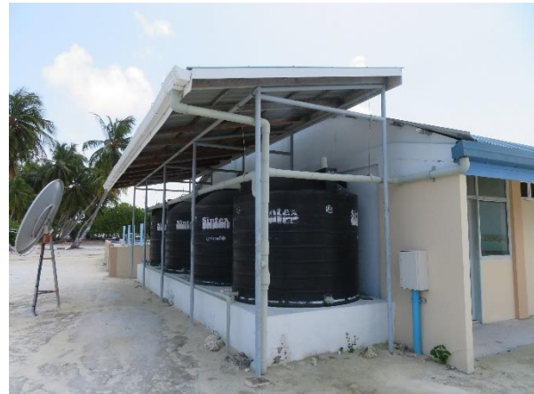
Figure 2.4.7 Rain Water Storage Tank in Maabaidhoo
