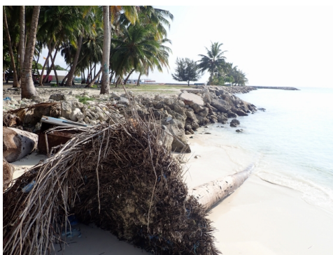
Figure 2.6.1 Coastal Erosion at the Down Drift Side due to Port Construction
