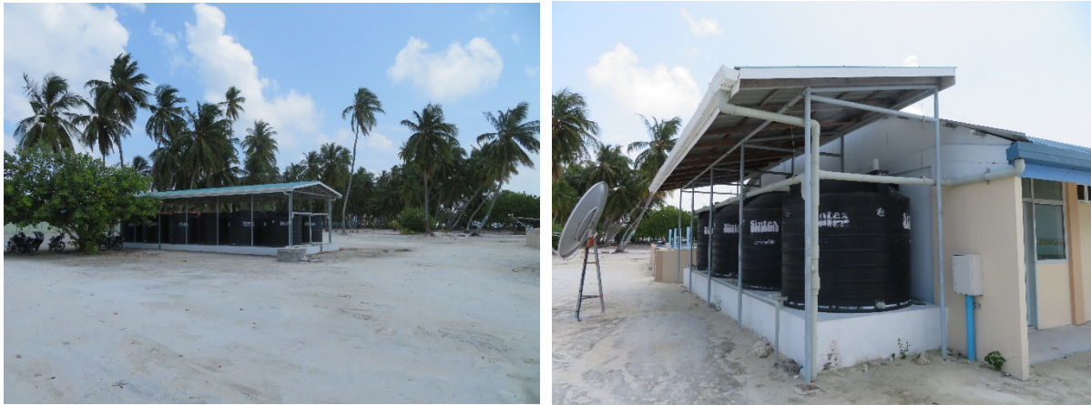
Figure 2.4.7 Rain Water Storage Tank in Maabaidhoo
