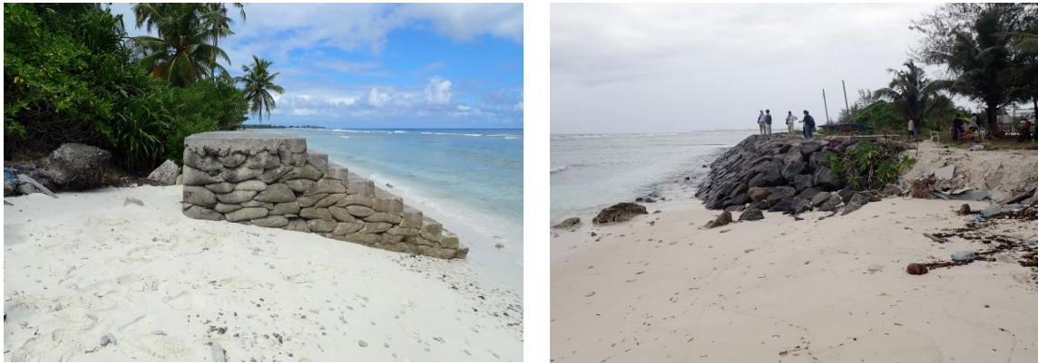
Figure 2.6.6 Construction of Revetment on Foreshore Area (Meedhoo in Addu Atoll)
