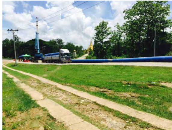
48" Dia; Transmission pipe(HDPE)
