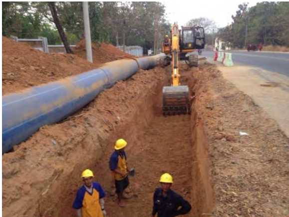
48" Dia; Transmission pipe(HDPE)
