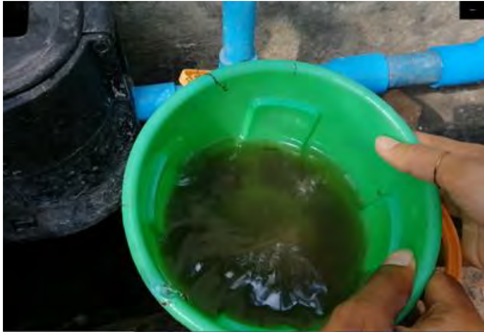
Water quality from house connection pipe line
