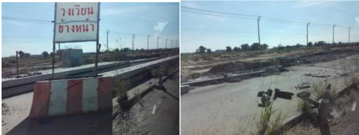
Investigation at the project Rom Klao Bridge
