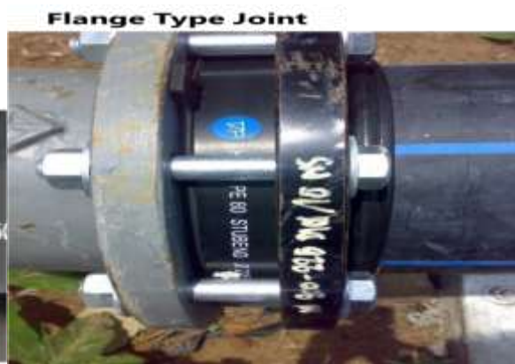
HDPE Flange Type Joint
