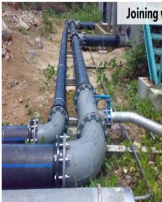
Joining with HDPE
