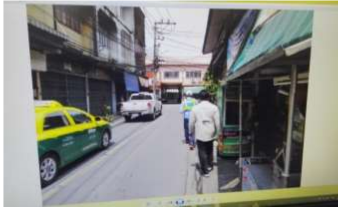
Closely Located Electricity Pole, Residence and Road
