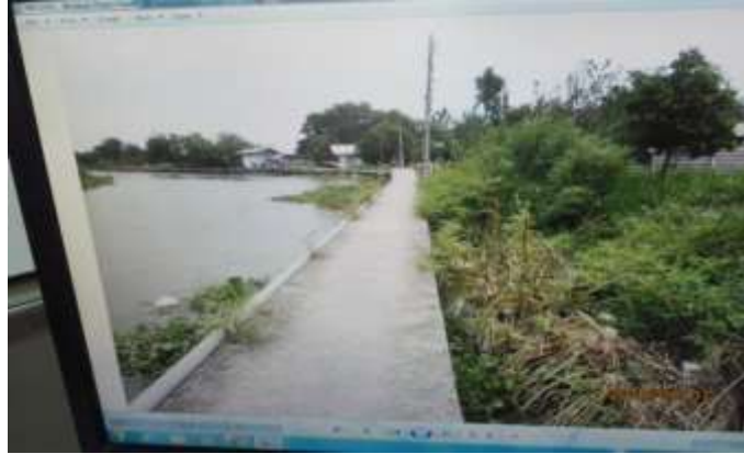
Pipe laying on the concrete road constructed over the creek
