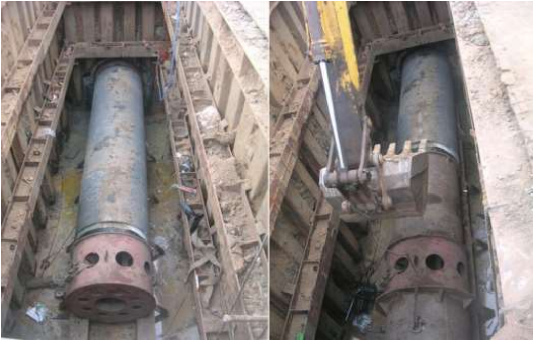
Dummy Pipe is inserted.
