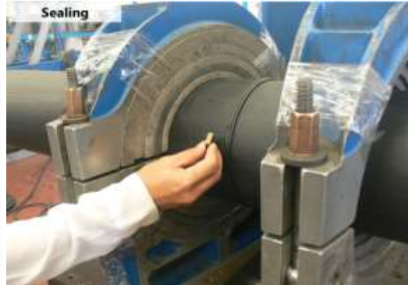
HDPE Flange Type Joint
