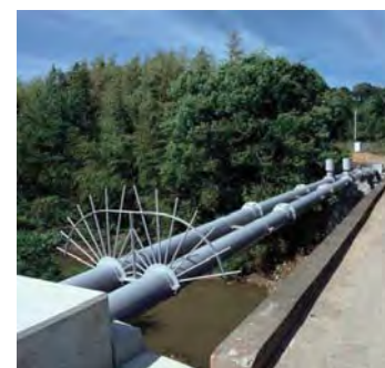
Water pipe bridge
