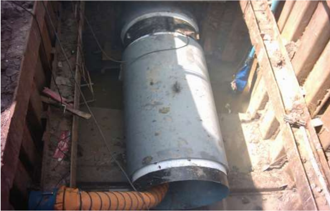
Welding Joint are checked by X-Ray Test.
