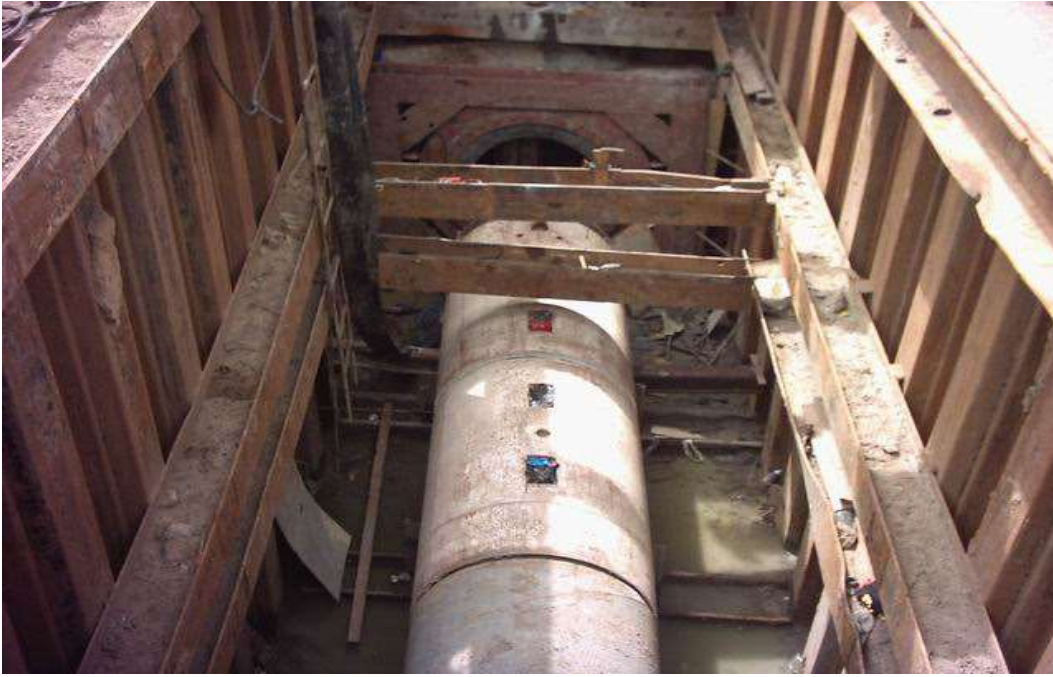
Dummy Pipe is inserted.
