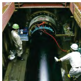
Pipe-in-pipe method
