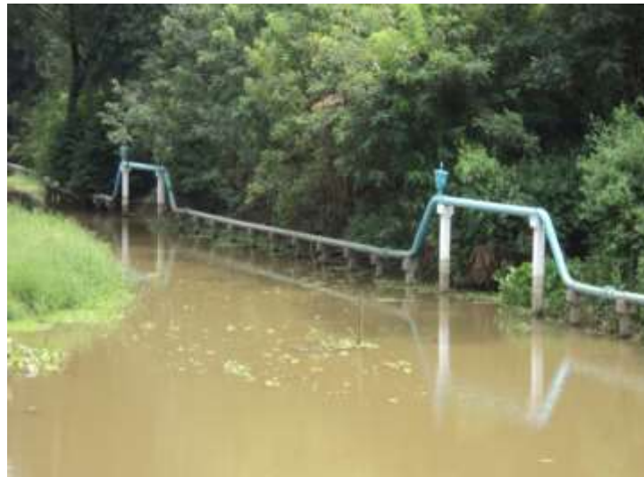
Usage of bends at the junction of creeks and channel
