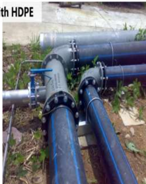
Joining with HDPE
