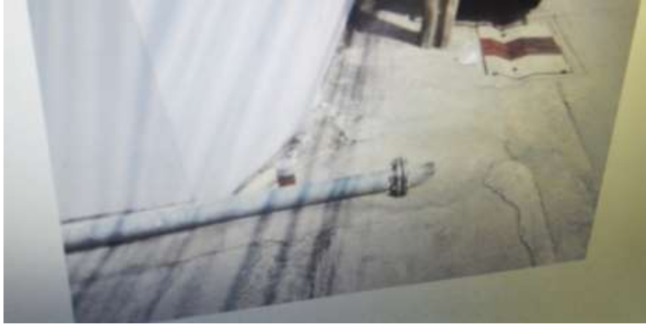
Unsystematic Pipe Connection
