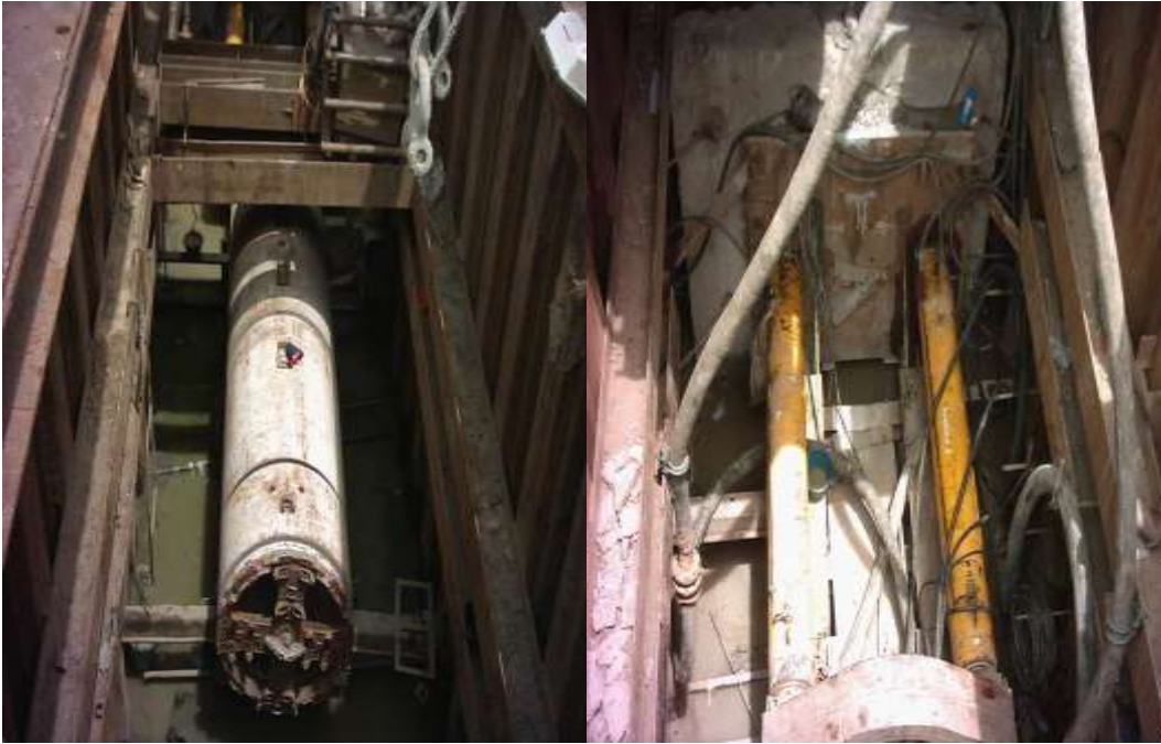
Earth Pressure Balance weight and Jack Machine are used in Jacking.
