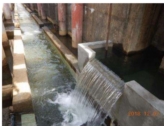
Raised outflow weir (Phase 1 pilot filter)
