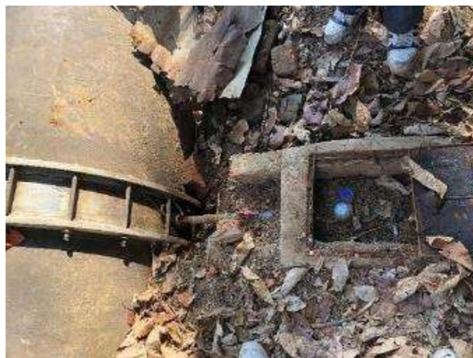
Photo 2-37: Direct branching from transmission main
