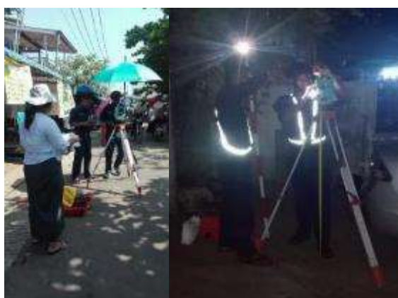
Photo 2-45: Topographical survey by total-station
