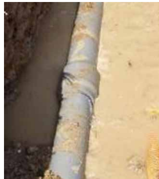
Situation of a leak
