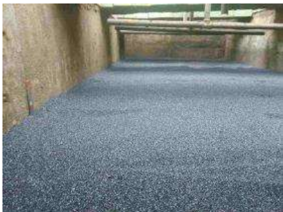
Replaced anthracite (Phase 2 pilot filter)
