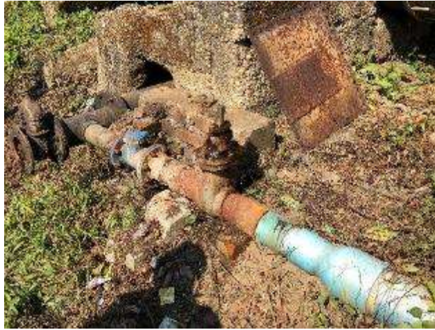
Photo 2-58: Damaged meter near the Gyobu transmission pipe
