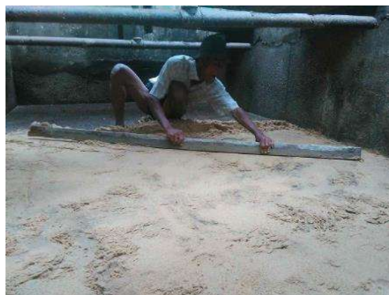
Replaced filter sand (Phase 2 pilot filter)
