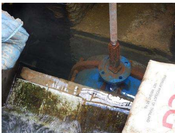
Replaced effluent valve (Phase 1 pilot filter. The weir is before improvement)
