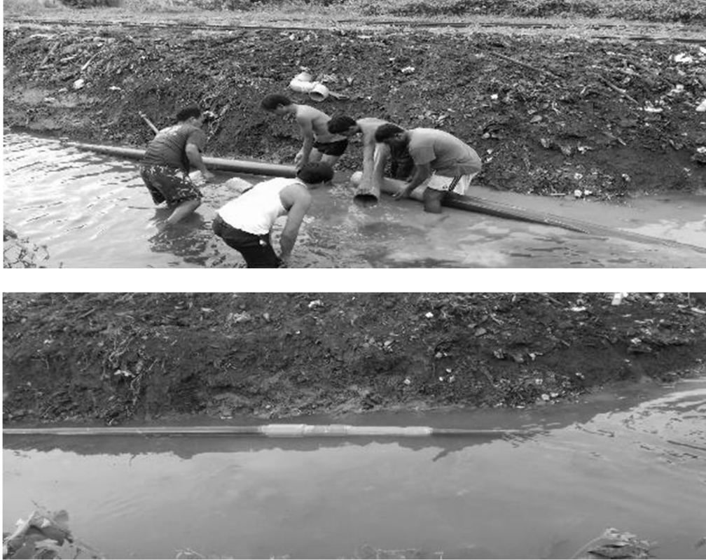
Photo 2-35: Leakage repair work in a creek
