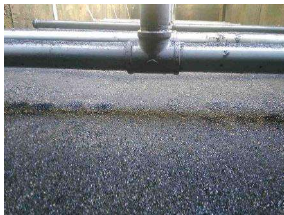
Newly set surface wash nozzle (Phase 2 pilot filter)
