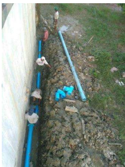
Photo 2-70: New desludging pipes equipped in No.1 sedimentation basin of Phase 1 (Outside of the basin)
