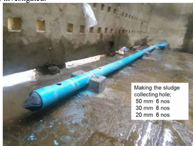
Photo 2-69: New desludging pipes equipped in No.1 sedimentation basin of Phase 1
