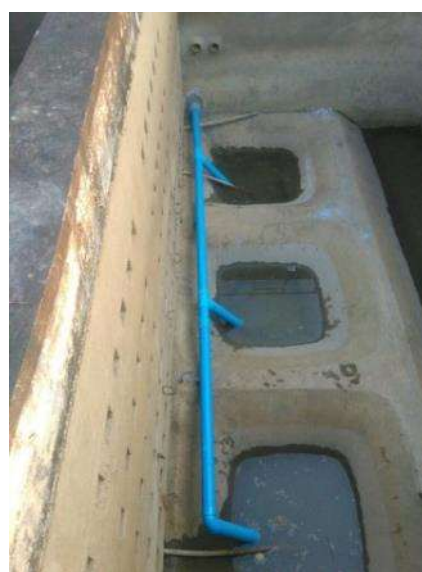
Photo 2-71: Replaced desludging pipes in No.1 sedimentation basin of Phase 1
