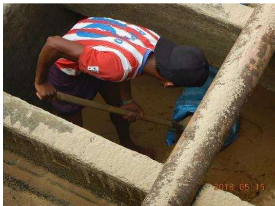
Replacement work of filter sand (Phase 1 pilot filter)
