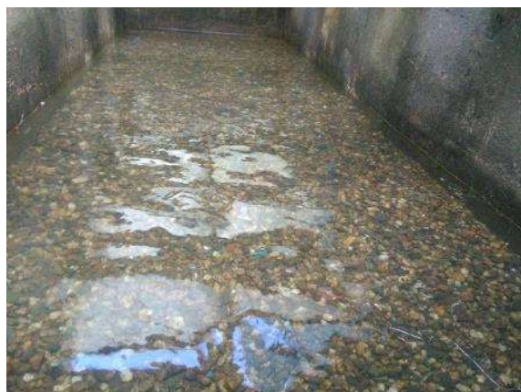
Replaced gravel (Phase 2 pilot filter)
