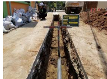
C/P learned backfill and construction photo
