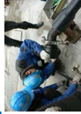
【Plumbing training for small bore diameter distribution pipes (φ100)】
