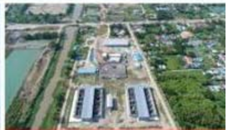
Lagunbyin Water Treatment Plant
