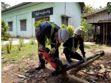
Pipe cutting training
