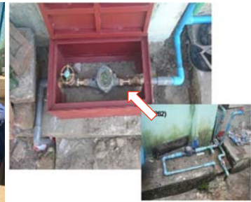
Install meter at proper location with meter box
