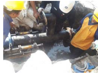
Connecting to existing distribution line
