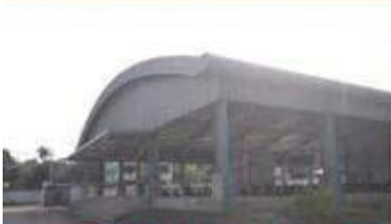
Training Yard at Yegu Pumping Station
