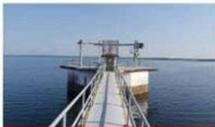
Intake Tower of PhuGyi Reservoir
