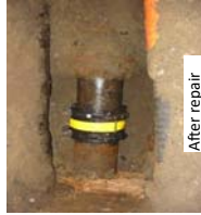
Splitting swivel joint ring
