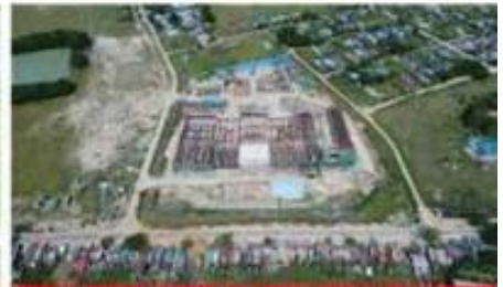
Service Reservoir for Zone (8) in Dagon Myathit (East) Township
