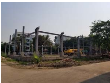
Foundation and framework construction
