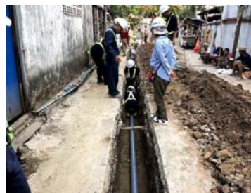
C/P trained piping work in trench (RRVP)
