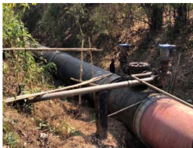
Direct branch situation from Gyobyu line
