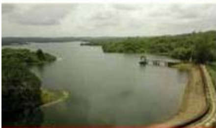
Intake Tower of Gyobyu Reservoir
