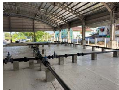
Piping work training field
