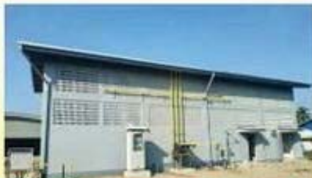
New Chlorination Facility at Yegu Pumping Station
