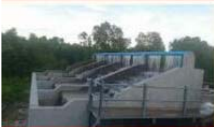
Iron Removal from the Groundwater by Aeration
