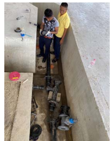
All pipes were installed by C/P
