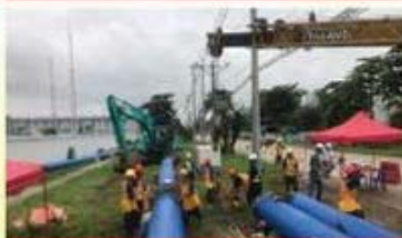
710mmØ HDPE Pipe laying in Thaketa Township
