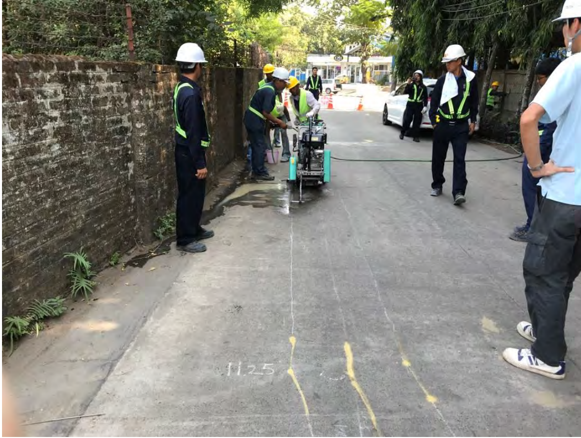
Pavement cutting
