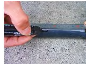
3- Insertion length marking
