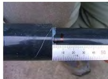
7- Check the insertion length
