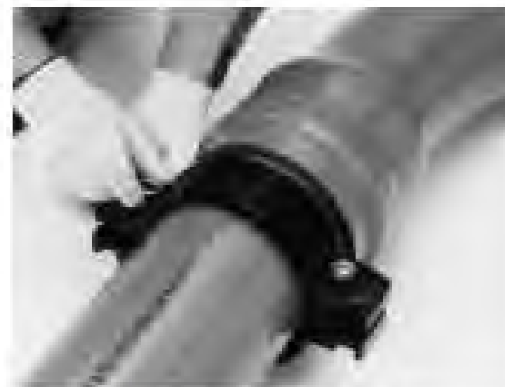
2. Partially tighten the spigot saddle
