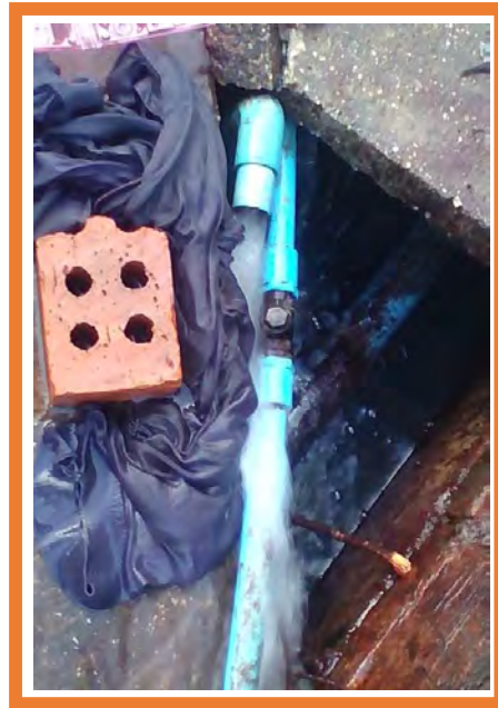
Leakage on service pipe
