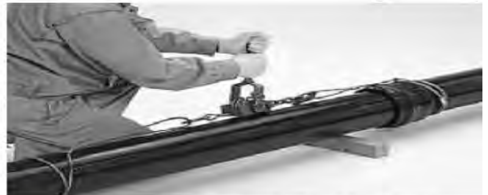
Insertion using a ratchet clamp
