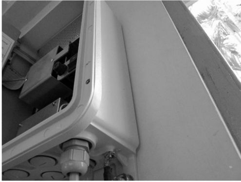
Installation of FG
