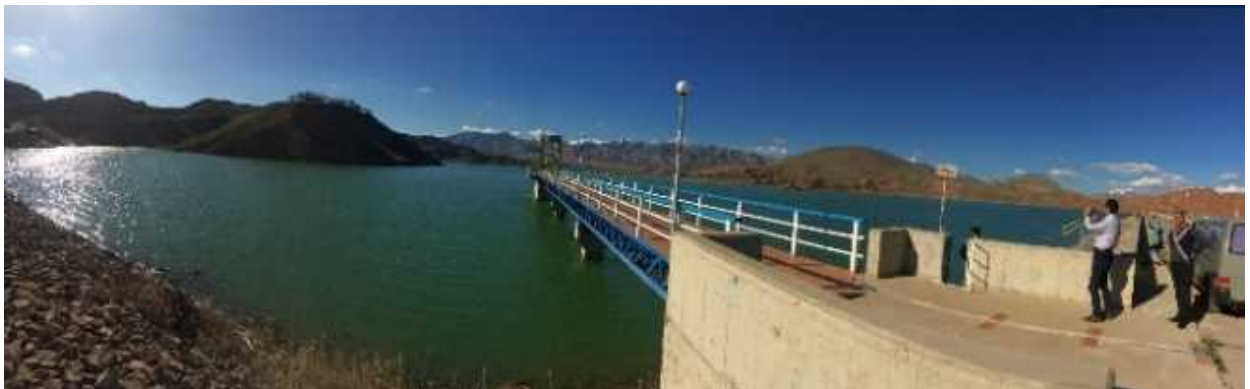
Nahand Dam (No. 4 in Figure 2.4.1 and No. 6 in Figure 2.4.2)
