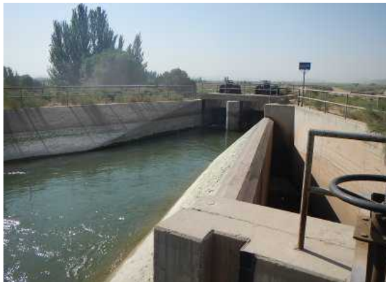
Main Irrigation Channel for Left Noruzlu Irrigation Network
