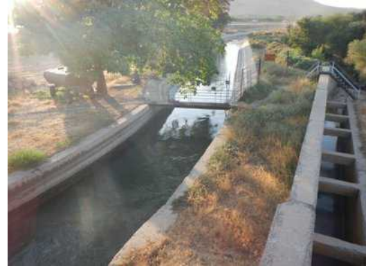
Irrigation Channel Nearby Inlet
