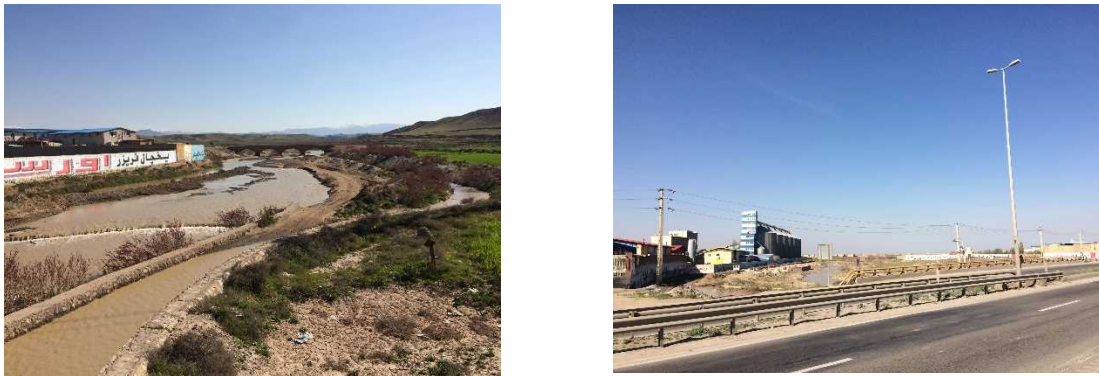
Pol Sanikh Hydrological Station (No.12 in Figure 2.4.1)
