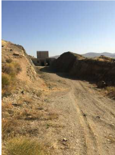
Simine Rud Dam (Inlet)
