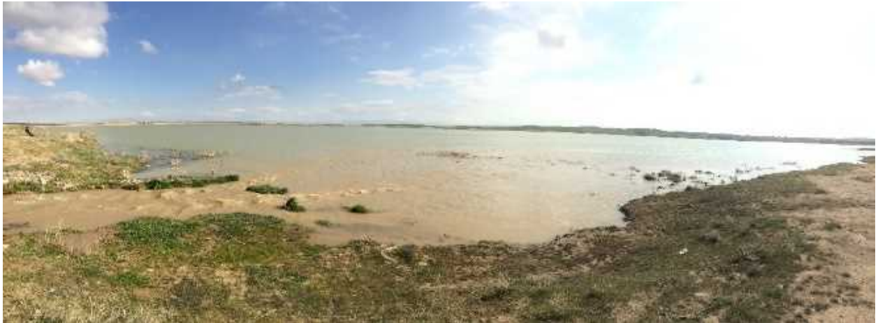
Kordikandi Dam (No. 2 in Figure 2.4.1 and No. 12 in Figure 2.4.2)
