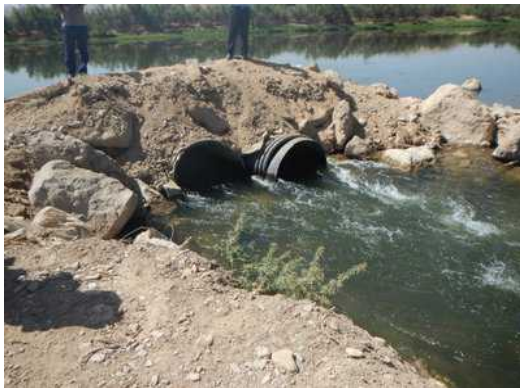
Inlet with concrete pipes
