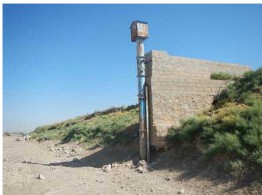
Simine Rud Hydrological Station
