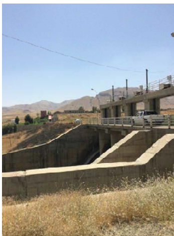
Zola Diversion Dam
