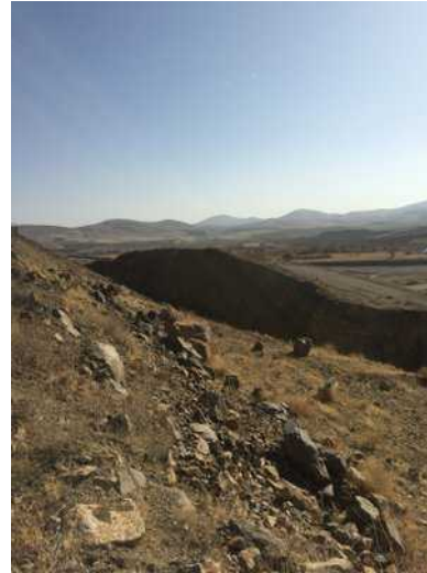
Simine Rud Dam (Dam Site)
