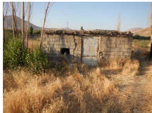
Well located nearby Adinan Hydrological Station
