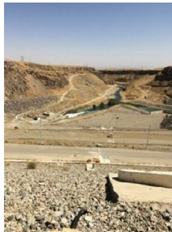
No. 1 Release of Water from Gate
