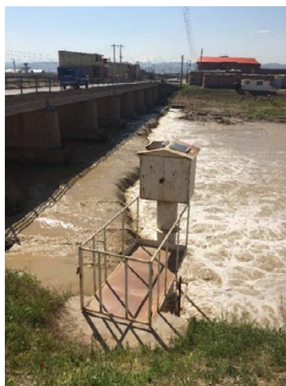
Akhola Hydrological Station (No. 10 in Figure 2.4.1)
