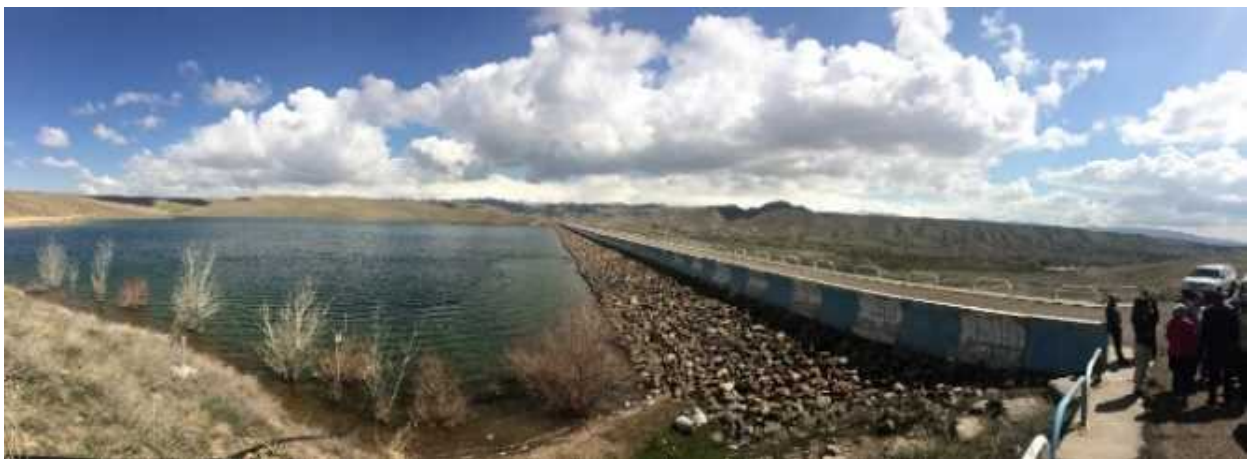
Tajiyar Dam (No. 3 in Figure 2.4.1 and No. 3 in Figure 2.4.2)
