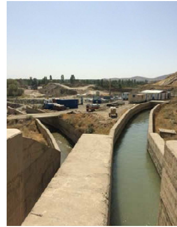
Main Channel for Balo Irrigation Scheme
