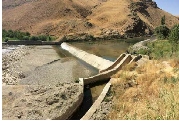
No. 19 Mobarak Abad Diversion Dam
