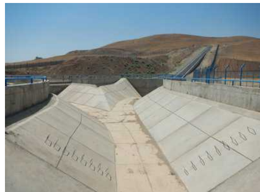
Jaldian Channel (Under Construction)
