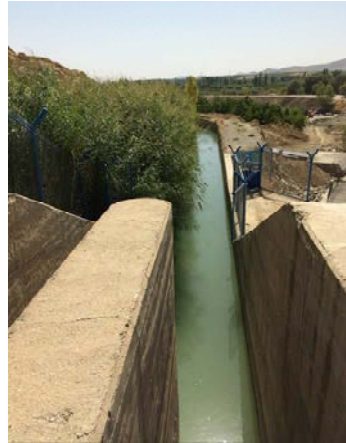
Main Channel for Dalmag Irrigation Scheme
