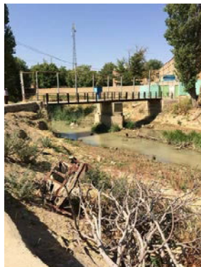
No. 18(1) Kashtiban Hydrological Station
