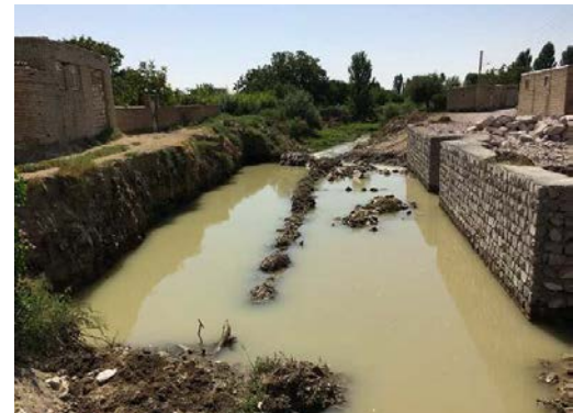
No. 18(2) New Construction Site of Kashtiban Hydro Station.
