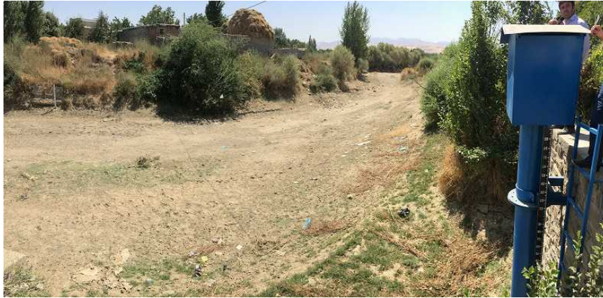
No. 24 Badarud Hydrological Station
