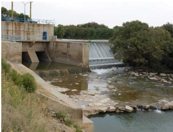
Weir Body of Dam
