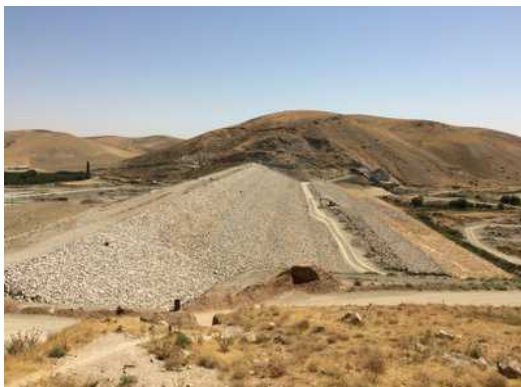
Chapar Abad Dam (Under Construction)
