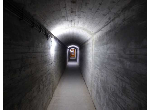
Accessway inside weir body
