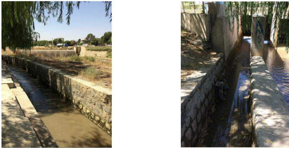
Figure 2.3.12 Emam Zadeh Diversion Dam (No. 25 in Figure 2.3.1)
