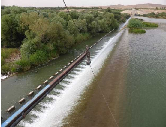
Overflow from weir (a view from the left bank)
