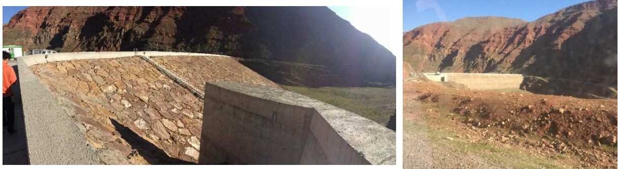
Figure 2.4.4 Shahid Madani Dam (No. 1 in Figure 2.4.1)
