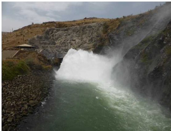
Release of Water from Gate
