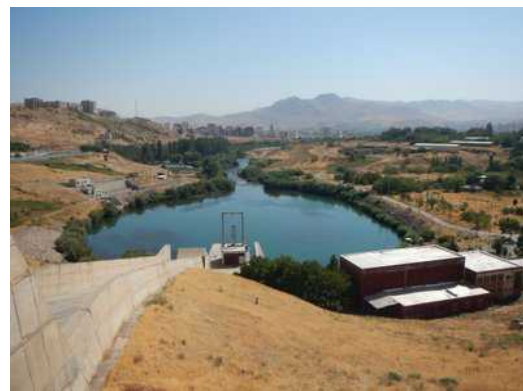
Mahabad Dam (Downstream of Weir)
