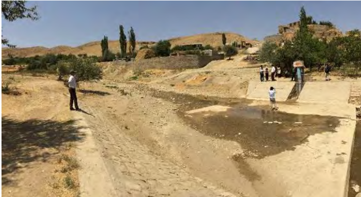
No. 12 Kalho Hydrological Station
