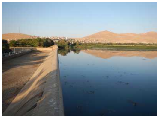
Yusef Kandy Diversion Dam
