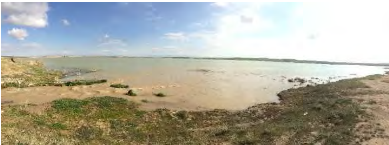
Kordikandi Dam (No. 2 in 図 2.4.1 and No. 12 in 図 2.4.2)
