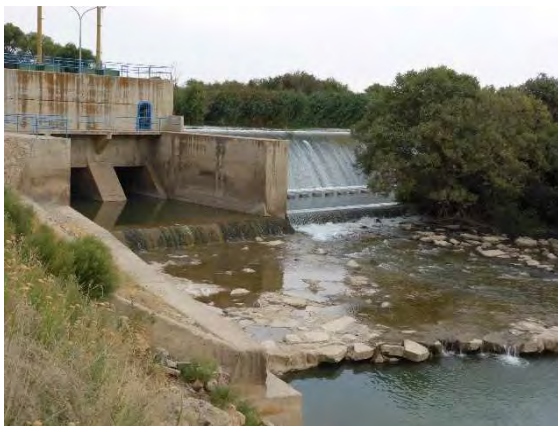
Weir Body of Dam
