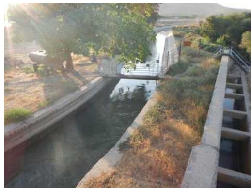
Irrigation Channel Nearby Inlet
