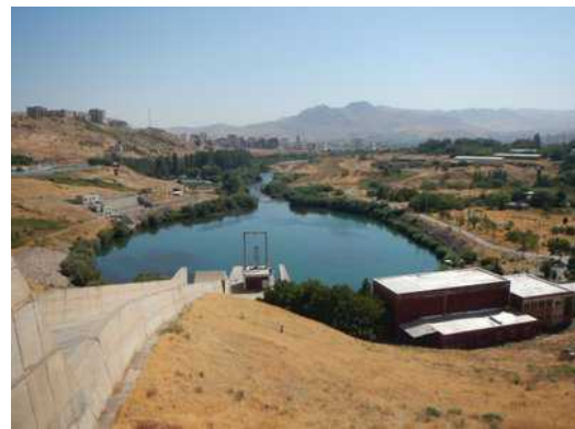
Mahabad Dam (Downstream of Weir)
