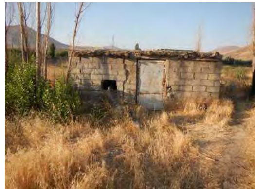
Well located nearby Adinan Hydrological Station
