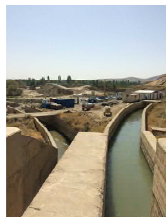
Main Channel for Balo Irrigation Scheme
