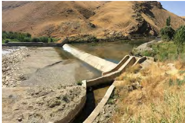
No. 19 Mobarak Abad Diversion Dam
