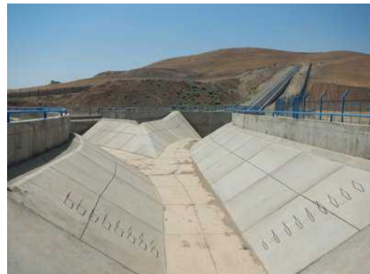
Jaldian Channel (Under Construction)
