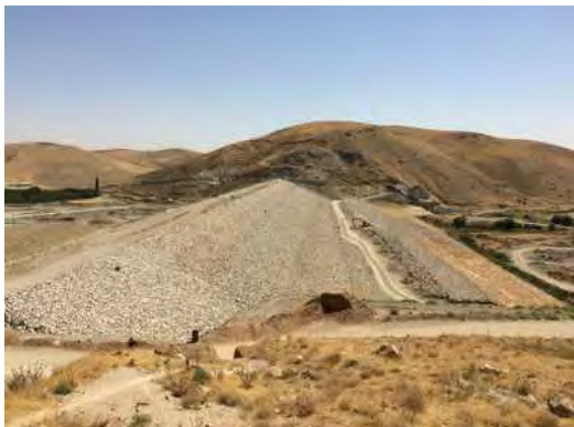
Chapar Abad Dam (Under Construction)
