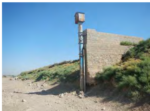
Simine Rud Hydrological Station
