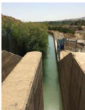
Main Channel for Dalmag Irrigation Scheme
