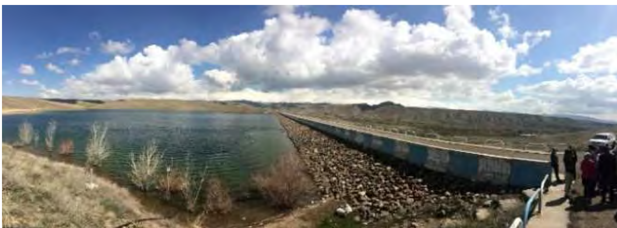
Tajiyar Dam (No. 3 in 図 2.4.1 and No. 3 in 図 2.4.2)
