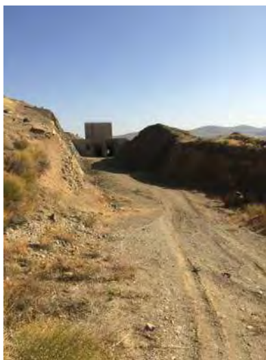
Simine Rud Dam (Inlet)
