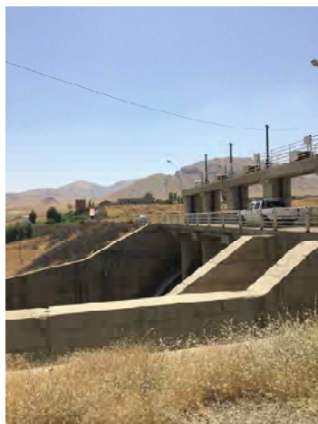
Zola Diversion Dam
