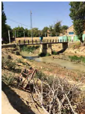
No. 18(1) Kashtiban Hydrological Station
