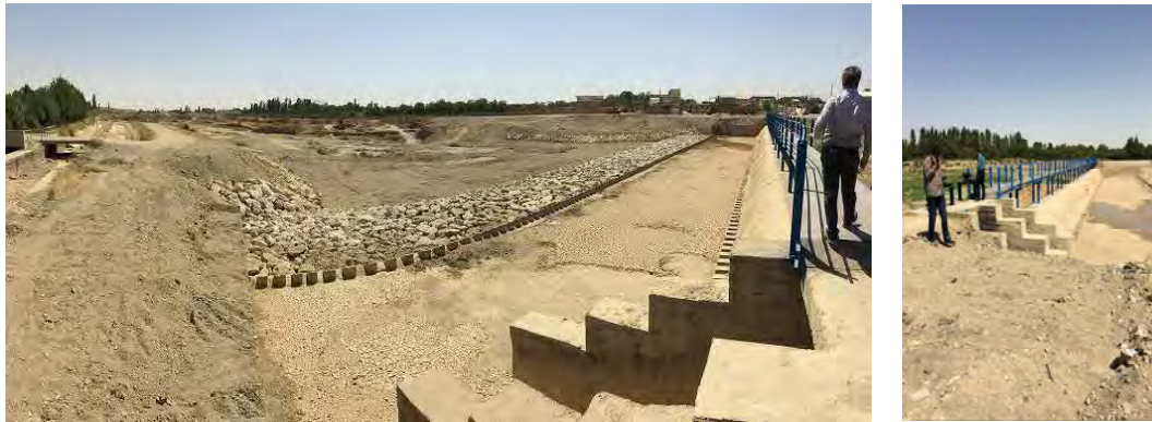
No. 8 Chongeralu Diversion Dam
